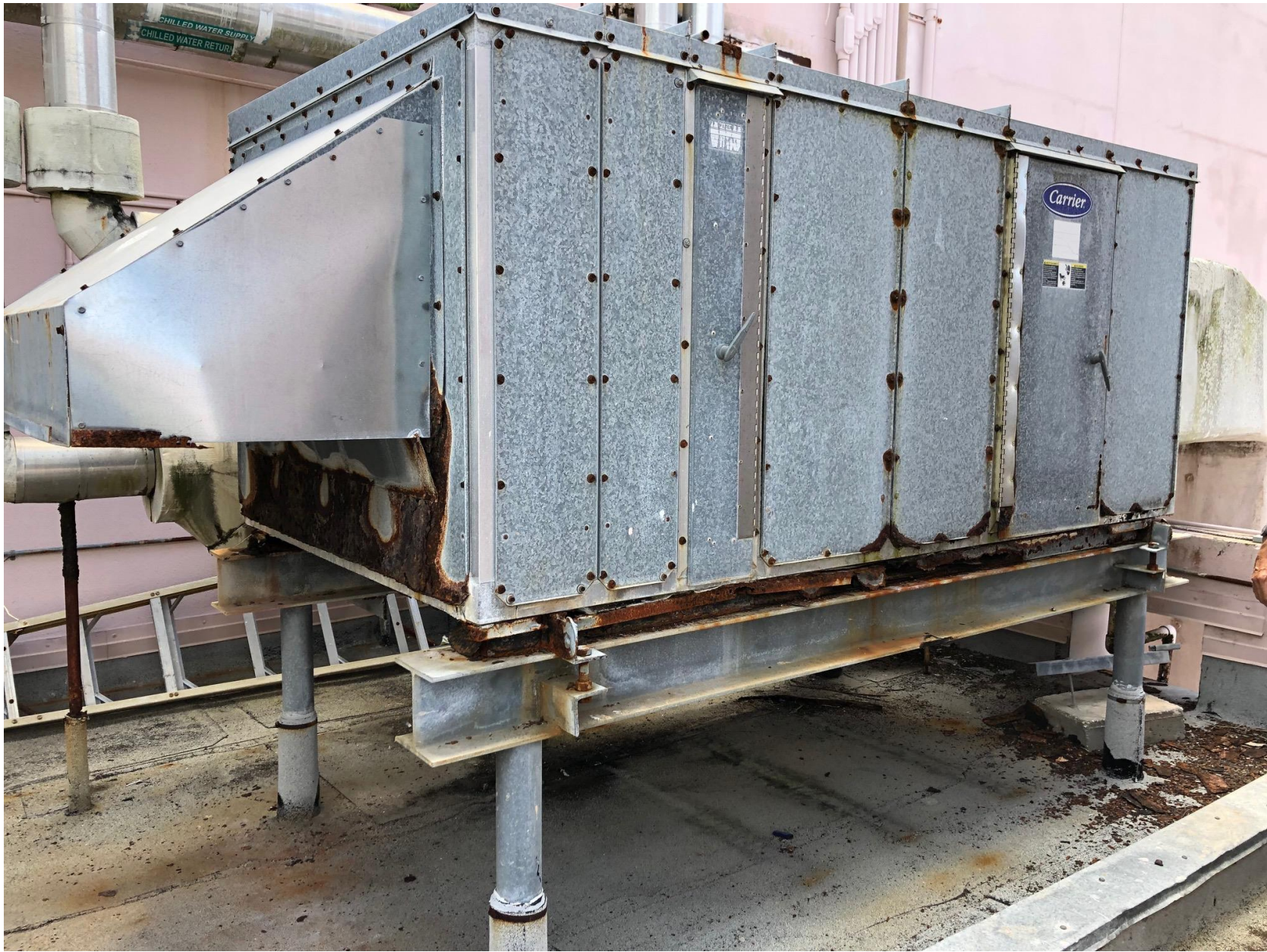
521 Thomas Street, Key west, Florida 33040 SITE VISIT
