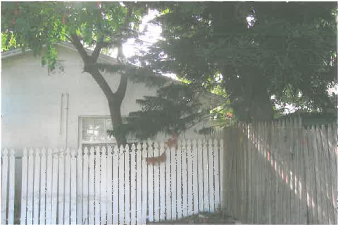
HOUSE ON LEFT SIDE
