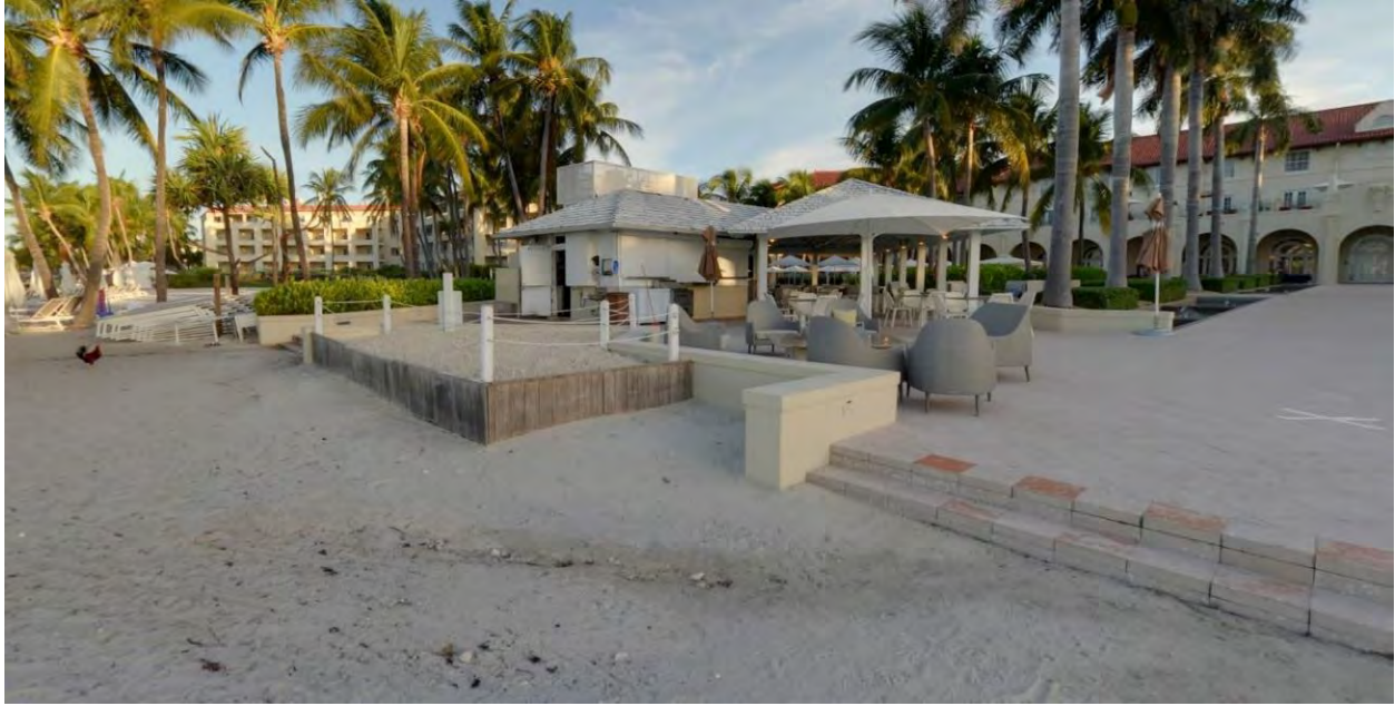
Photo depicting the west structure before demolition. The enclosed structure used to be the kitchen. Photo provided by applicant.
