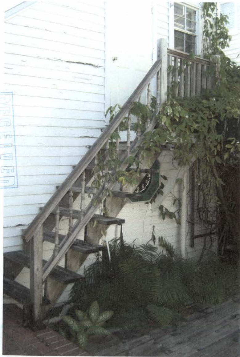
STAIR TO ROOM OVER GARAGE
