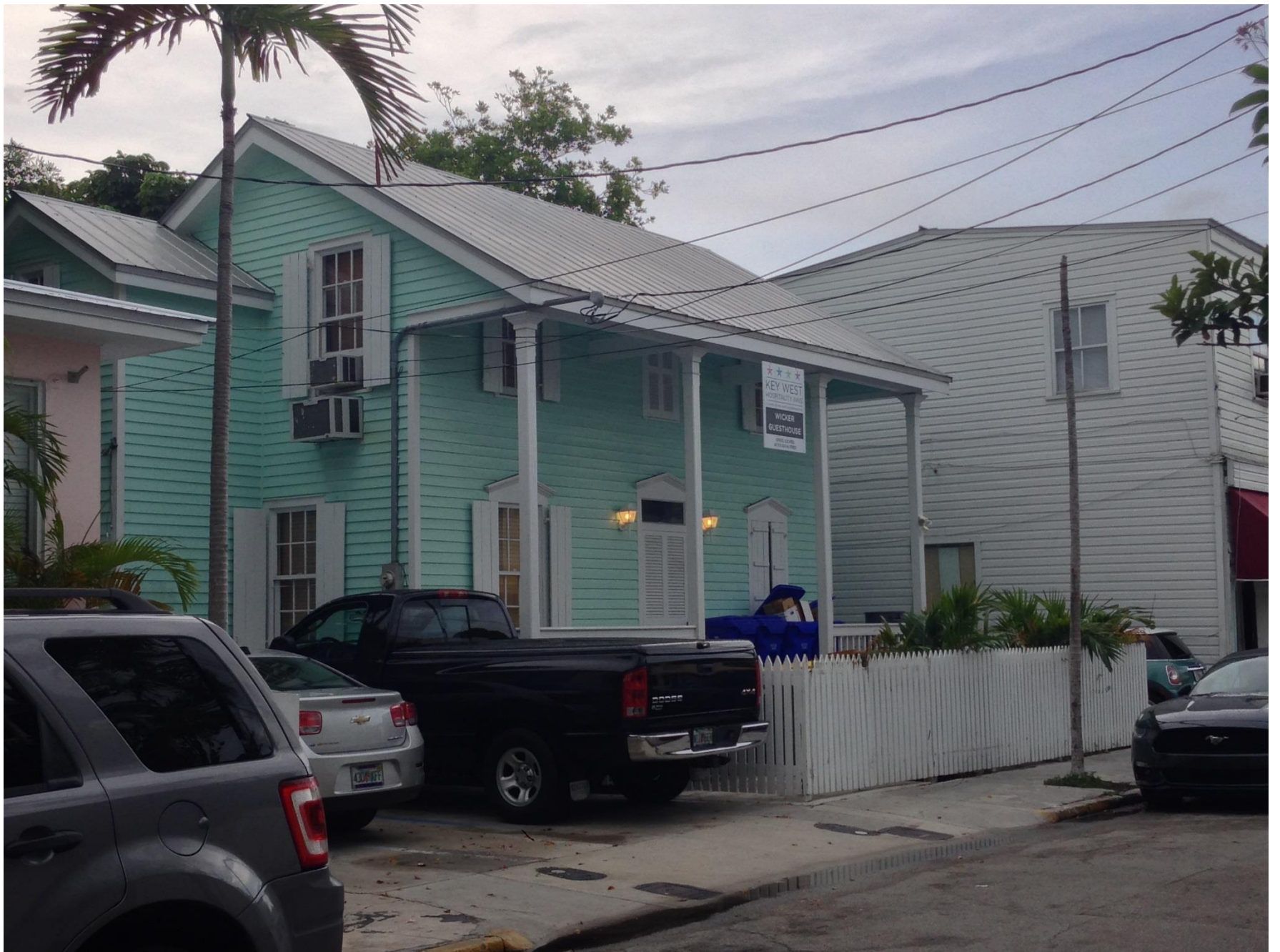
Eye-brow house at 508 Olivia. Note the four evenly spaced posts.
