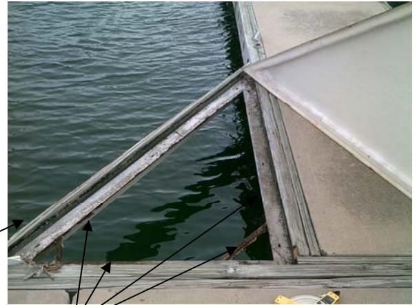
Bracing tri-frame to be replaced (4x 6' with 4' and 8' thru bolts/hardware)
