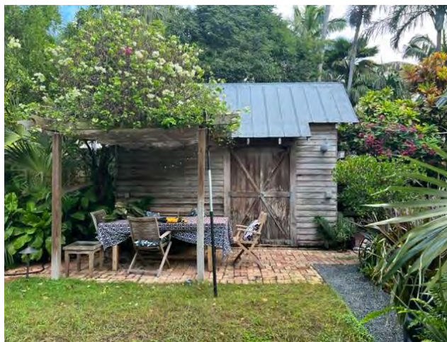
The accessory structure under review, existing.
