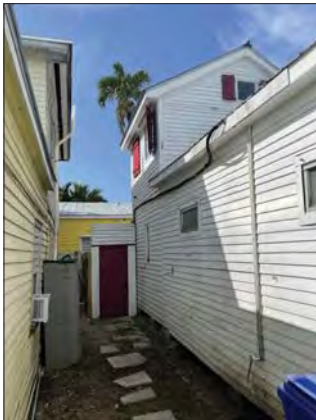
7 LOOKING SOUTH FROM EAST SIDE YARD
