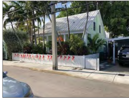
5 HOUSE ACROSS STREET LOOKING NORTH
