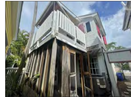
10 EXISTING REAR PORCH AND BALCONY
