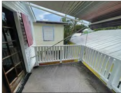
9 LOOKING EAST AND SOUTH FROM REAR BALCONY
