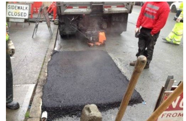
Temporary curb ramp along pedestrian detour
