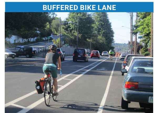
A bike lane with a painted buffer to increase space between bicycle riders and hazards such as passing traffic and car doors.
