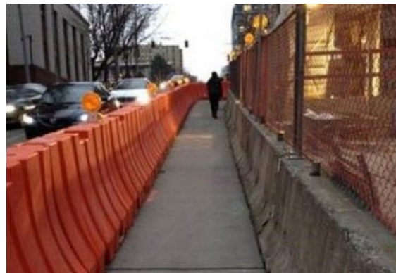
Pedestrian route adjacent to construction
