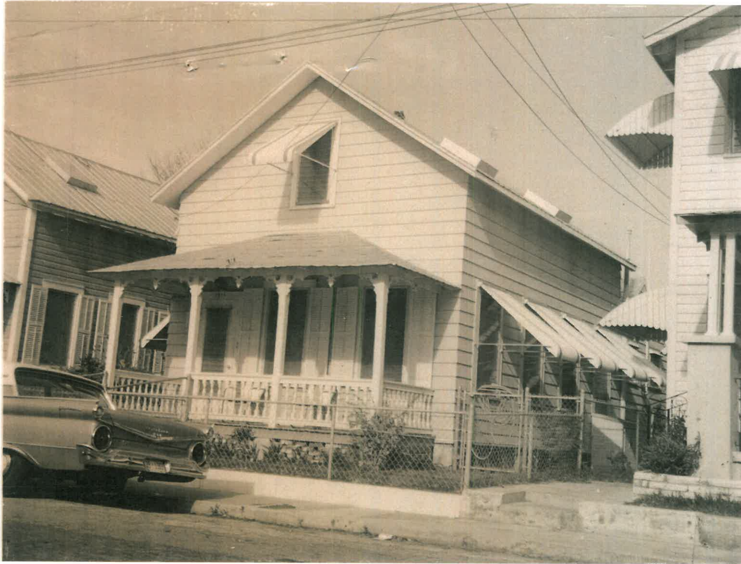
#1311 Pine Street photograph circa 1965 from the Property Appraisers office. Monroe County Library
