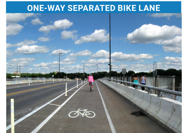
A one-way bike lane along a roadway vertically separated from motor vehicle traffic by a curb, flex-posts, and/or parking.
