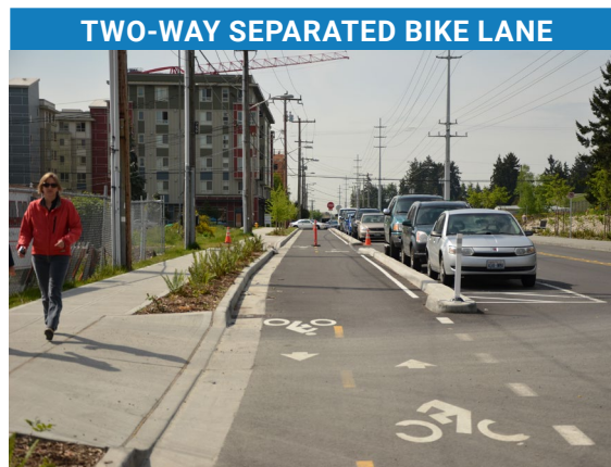
A two-way bike lane along a roadway vertically separated from motor vehicle traffic by a curb, flex-posts, and/or parking. May be at sidewalk level, street level or intermediate height.
