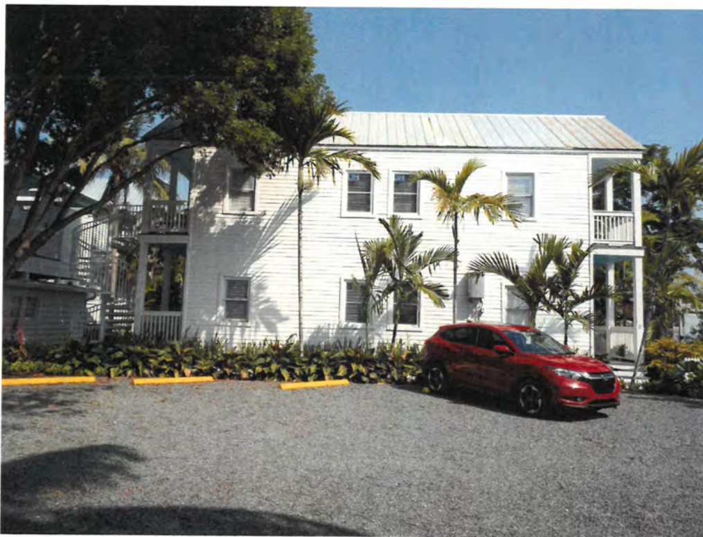
North - Rear View (opposite Truman Ave)
