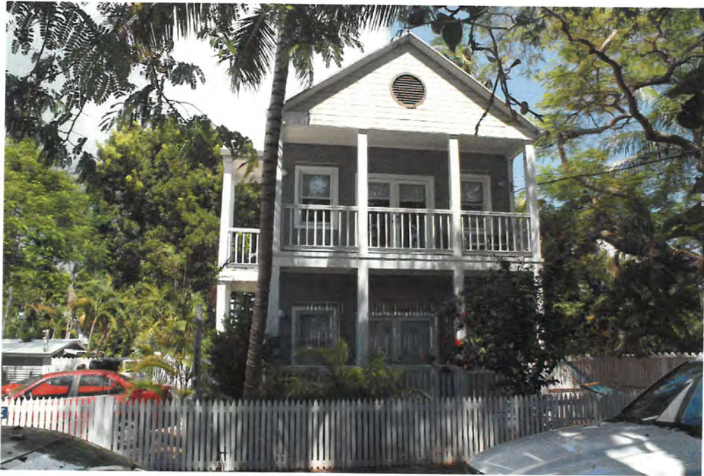
West - Before Construction
