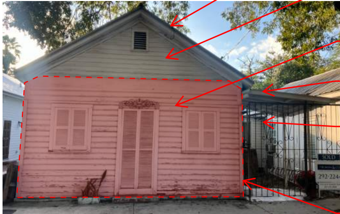
PHOTO 11: EAST WING FRONT ELEVATION
