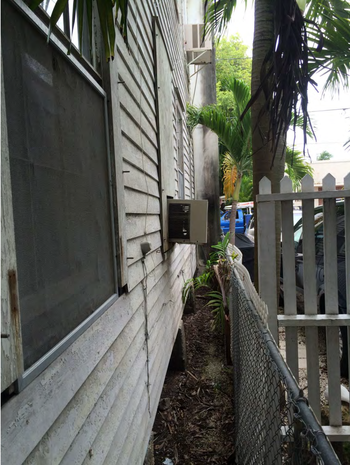
SIDE OF 421 SIMONTON LOOKING TOWARDS FRONT
