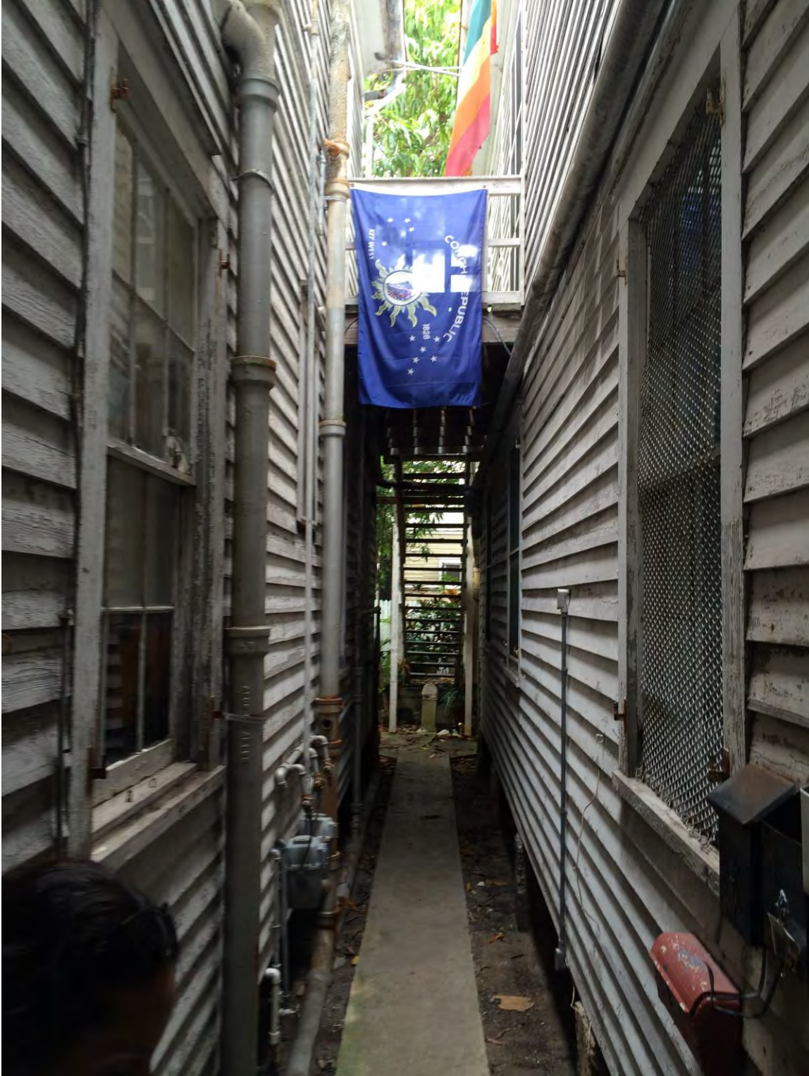
LOOKING TOWARDS THE REAR 421 AND 423
