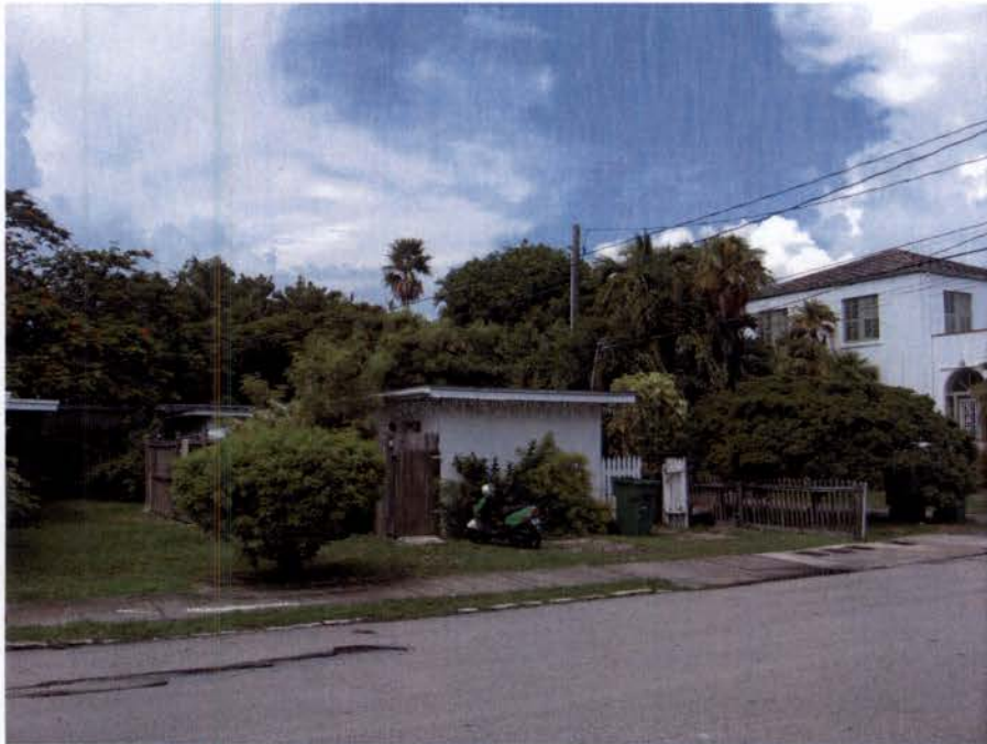
Adjacent building at 1506 Grinnell Street.
