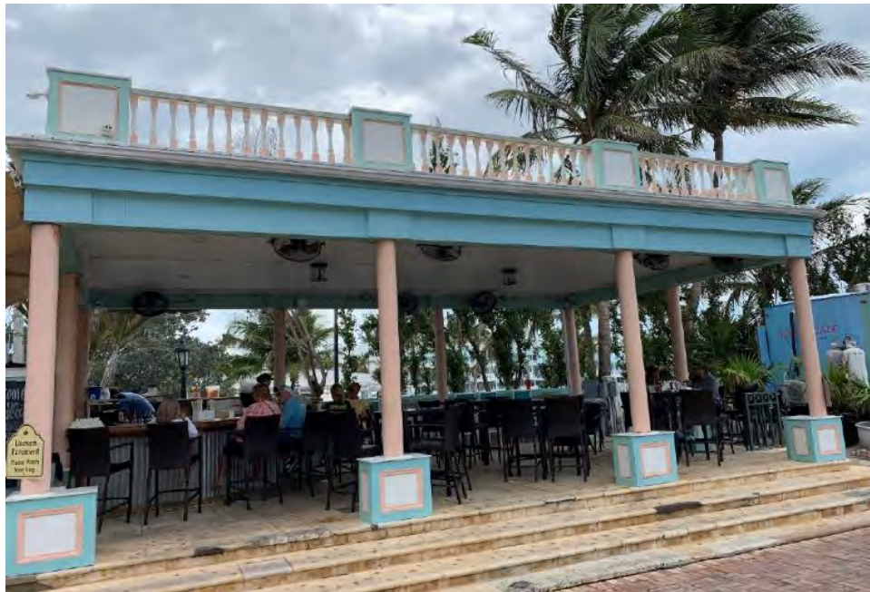
The accessory structure under review, existing.
