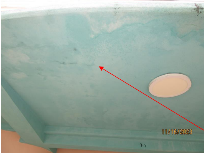
Front Entrance Roof
