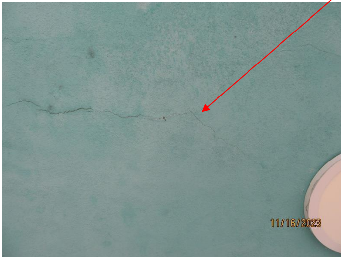
Front Entrance Roof
