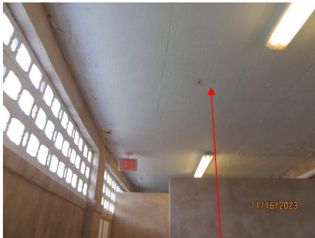
Men's Dressing Room Ceiling
