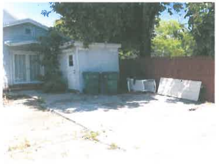
Shed and concrete to be removed
