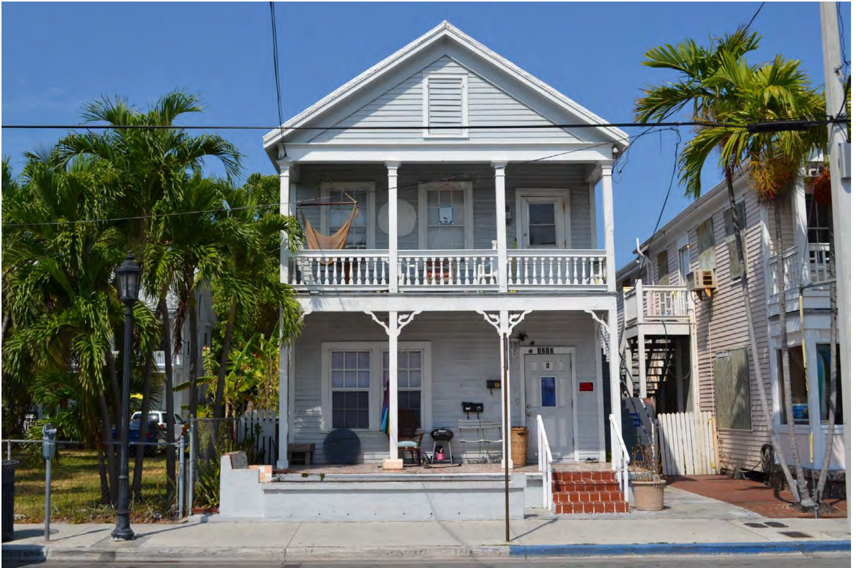
2011 Photo of 1212 Duval Street. Monroe County Public Library.
