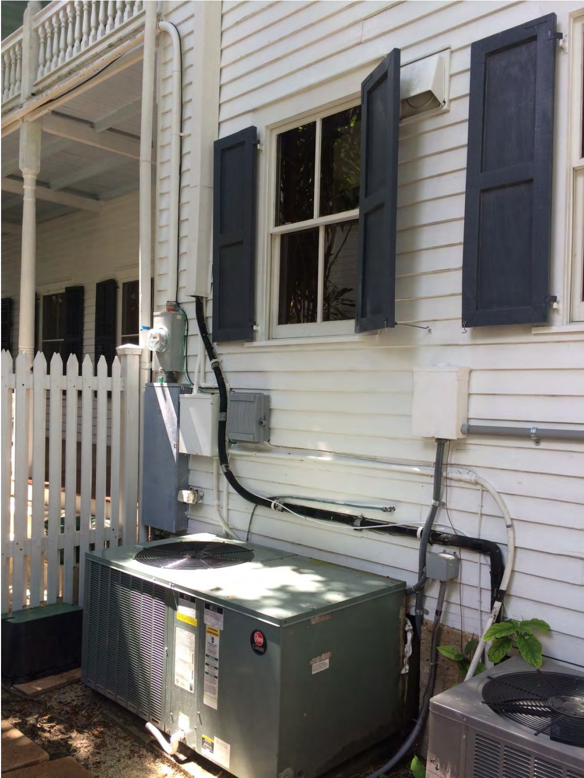
925 FLEMING STREET: SIDE OF HOUSE
