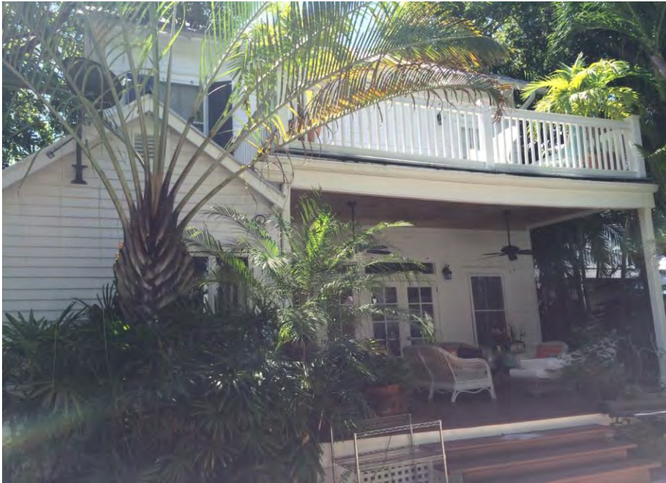
925 FLEMING STREET: BACK OF HOUSE
