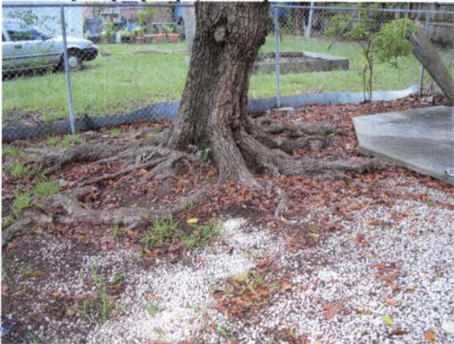
Roots of the Sapodilla Tree immediately in front of subject building.
