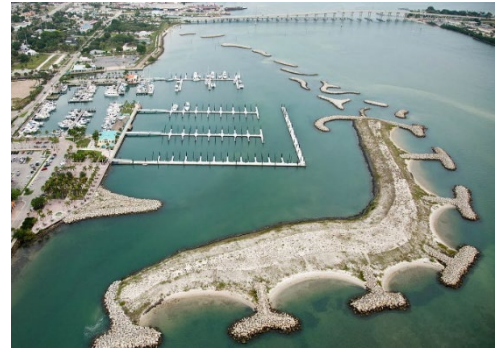
Fort Pierce Storm Protection Island, Tetra Tech
