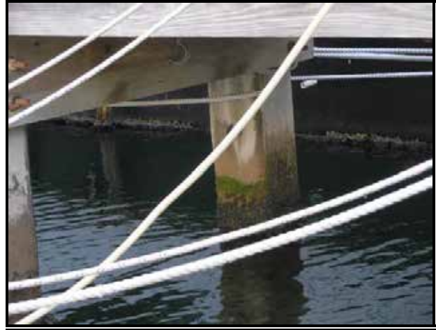
Wood deck and framing on concrete piles.
