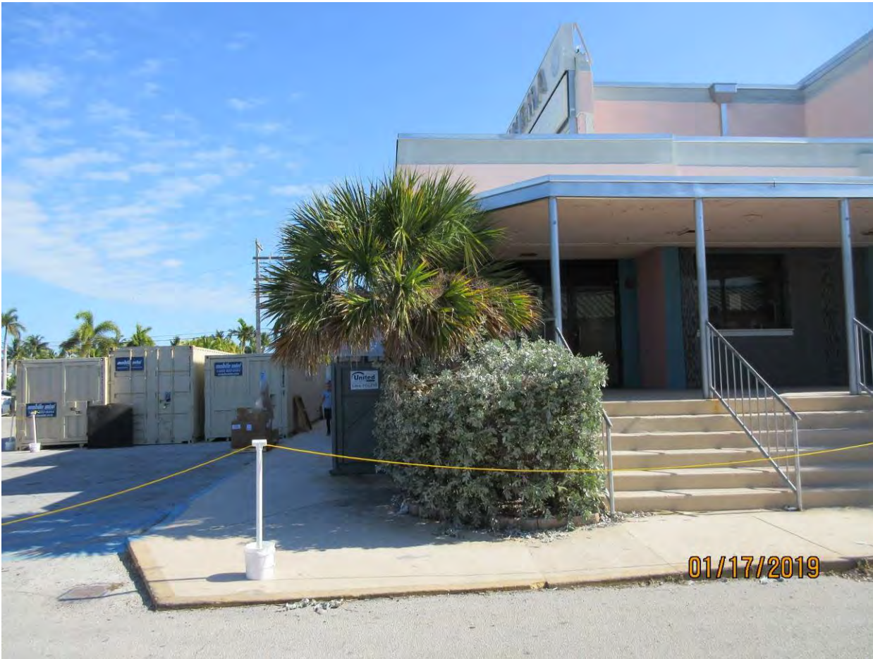
Entrance area: Sabal Palm to remain, silver buttonwood shrubs to be removed
