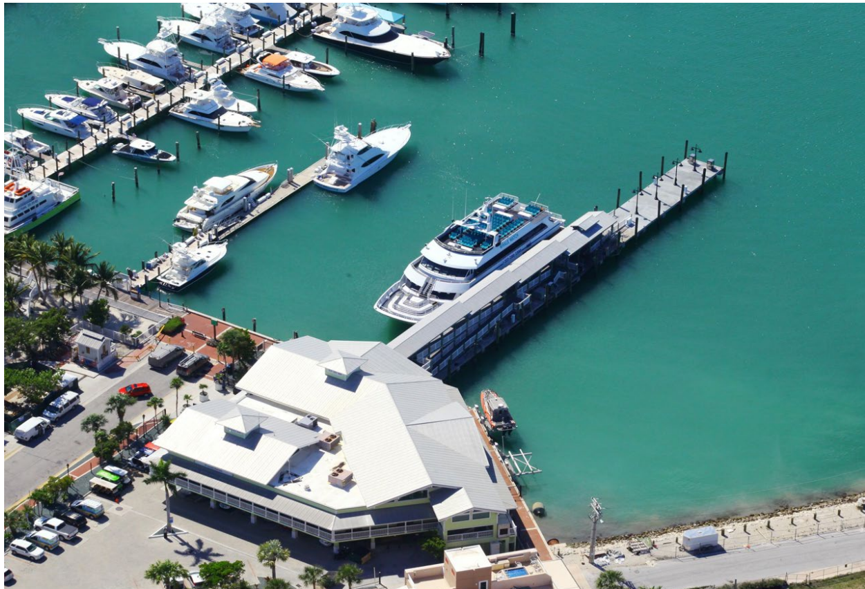
Insert 1: Existing Ferry Terminal Building, Pier, and Portion of Trumbo Road
