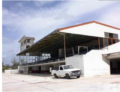
Asbestos testing at Old Dog Track, Stock Island
