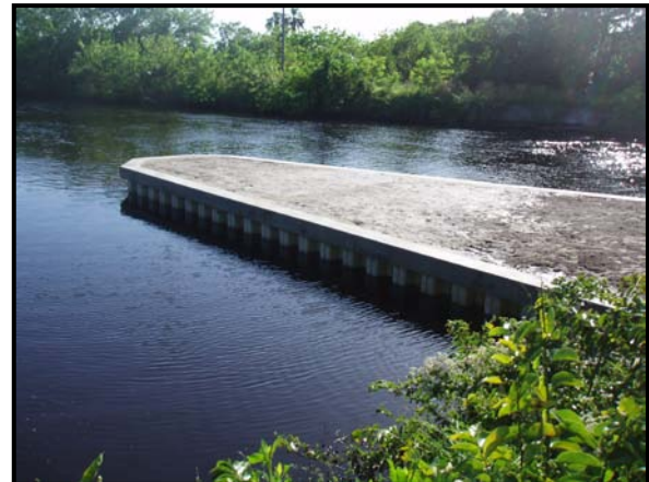
Shoreline with new seawall
