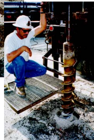
Test well drilling and soil testing for fuel tank removal and closure, Robbie's Marina, Stock Island
