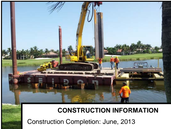
New vinyl seawall located on shoreline opposite littoral plantings. Note the tight working quarters between the new seawall and existing buildings.
