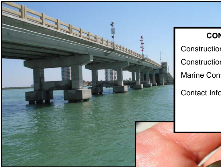
Big Carlos Pass Bridge
