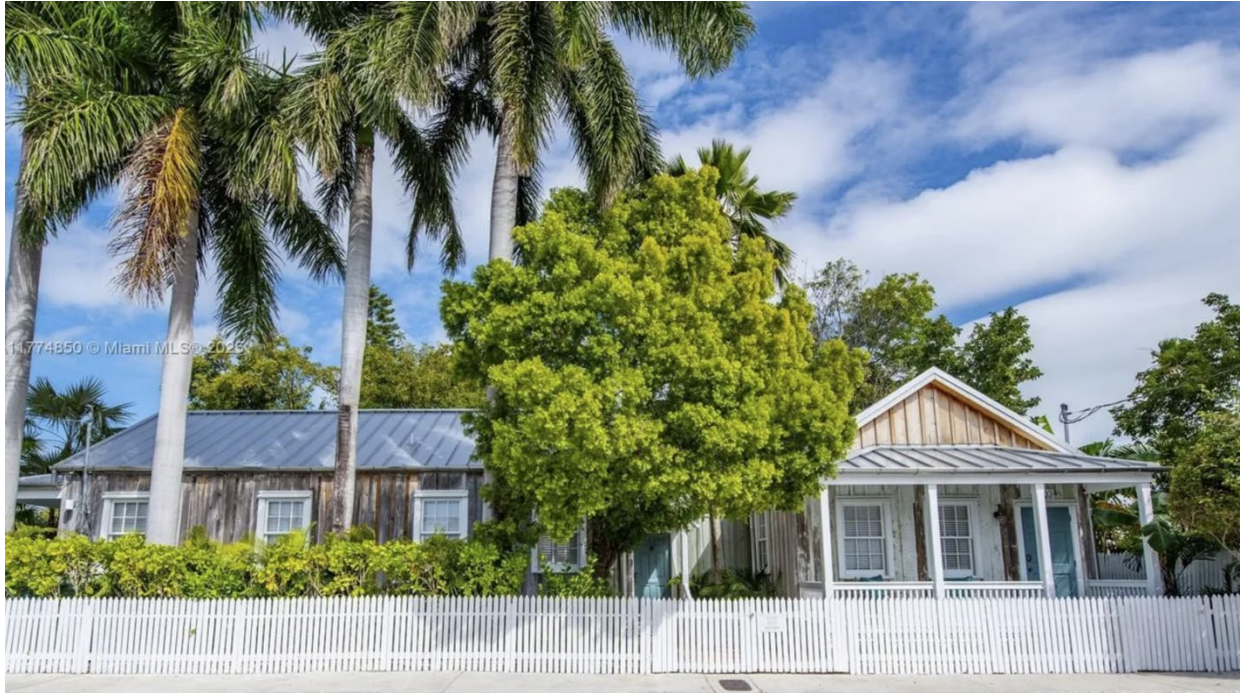
View of both houses on property from Florida Street.
