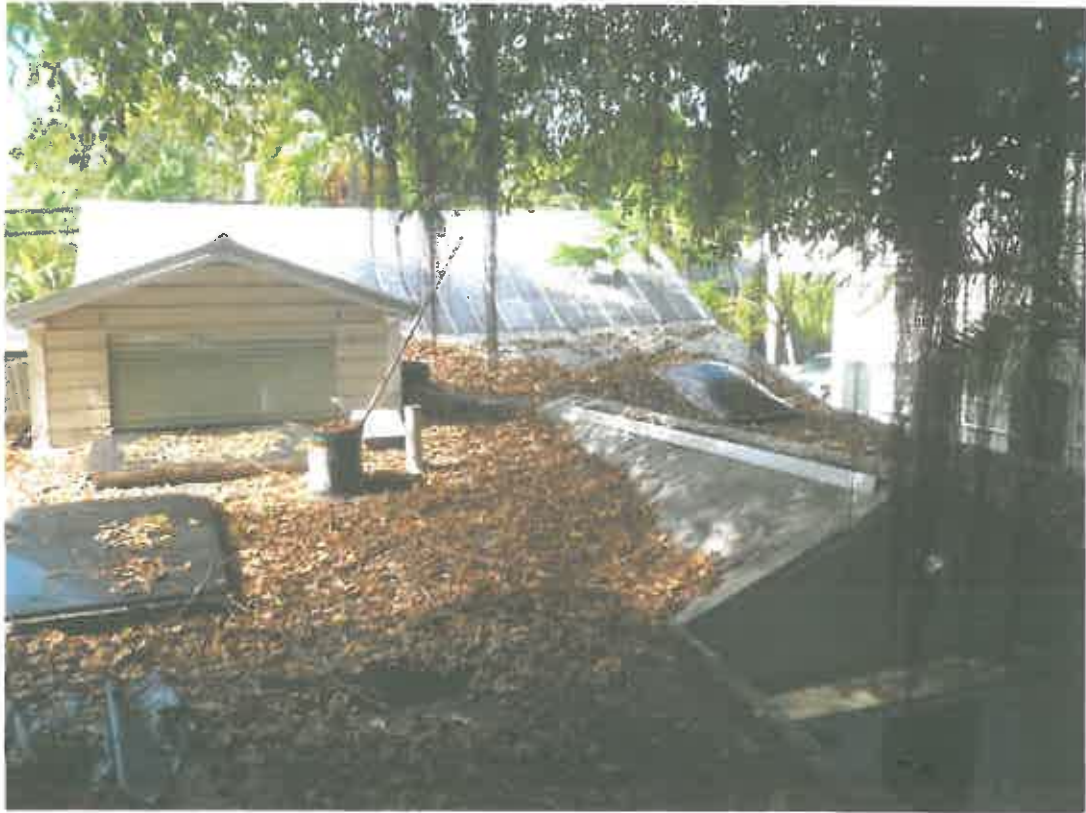
527 Margaret Street- View of roof from second story of rear addition
