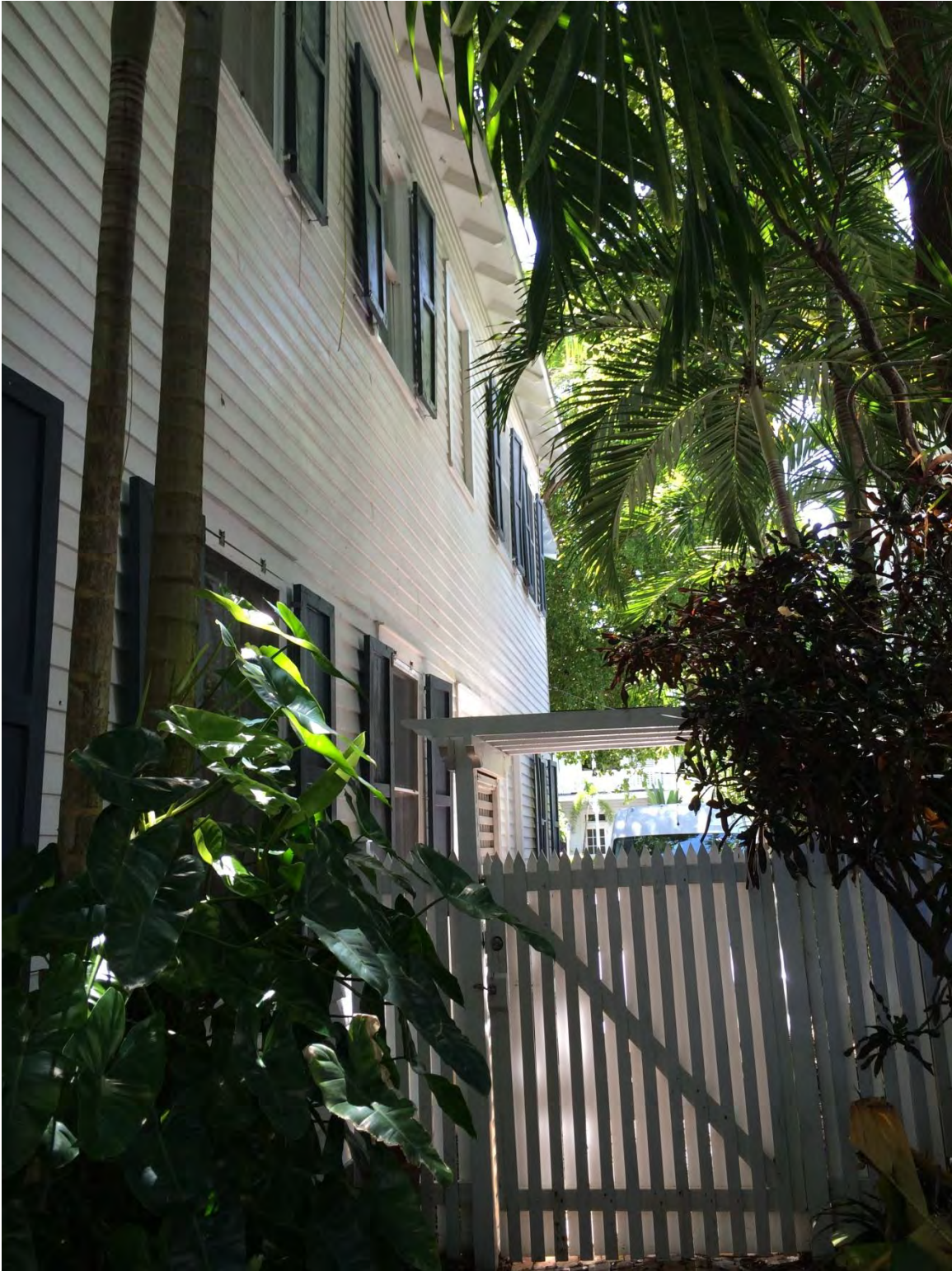
925 FLEMING STREET: SIDE OF HOUSE
