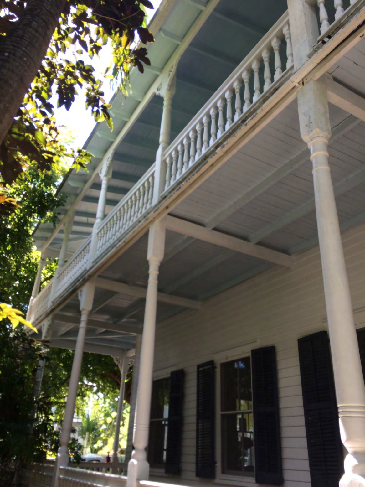
925 FLEMING STREET: SIDE OF HOUSE
