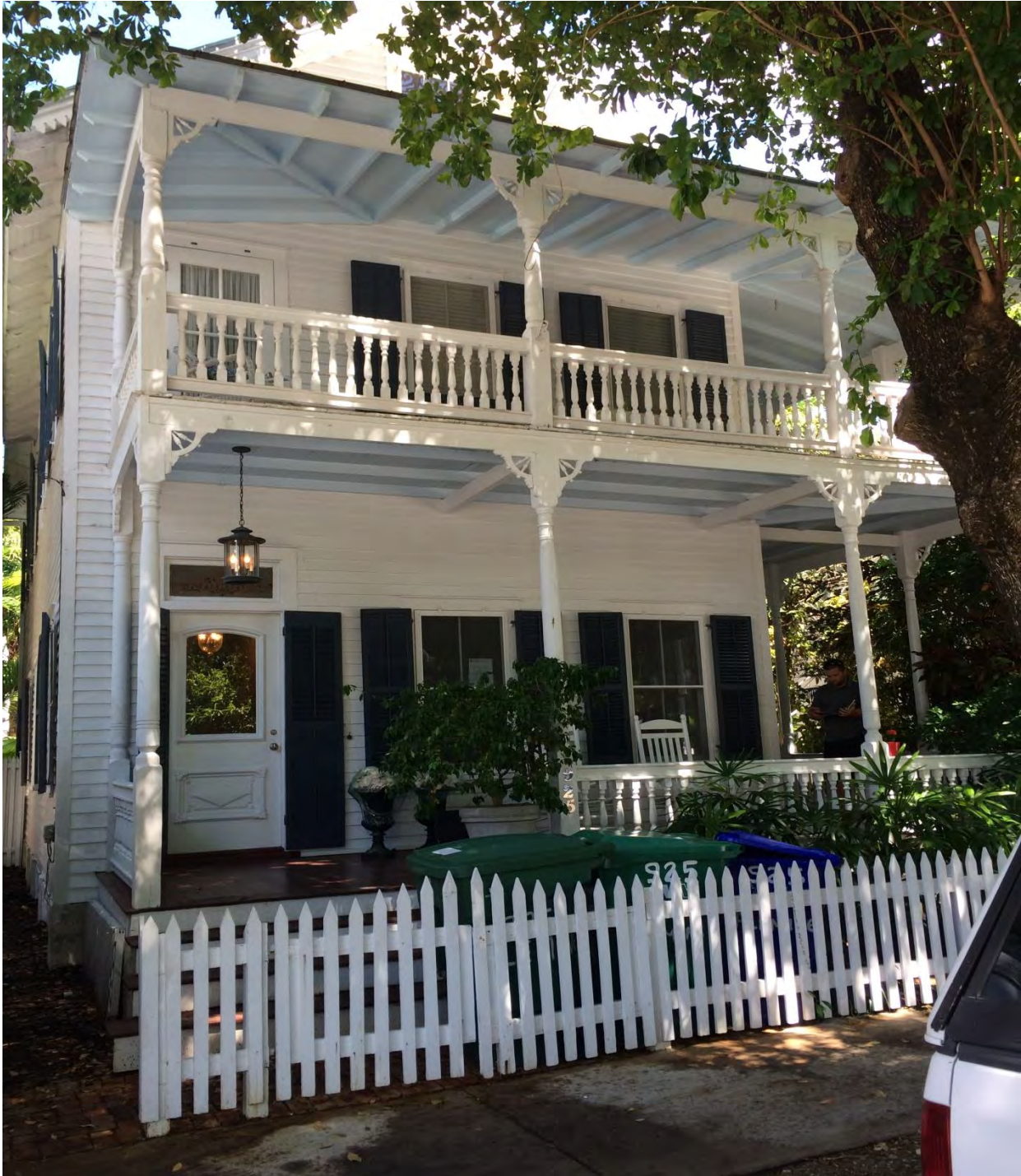
925 FLEMING STREET: FRONT OF HOUSE
