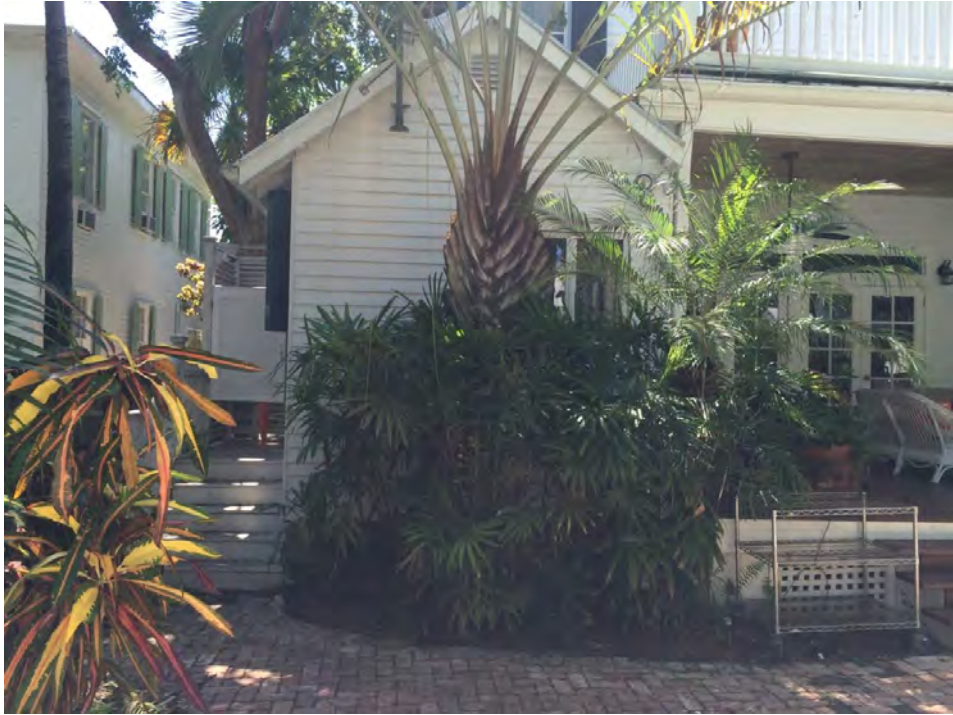
925 FLEMING STREET: BACK OF HOUSE
