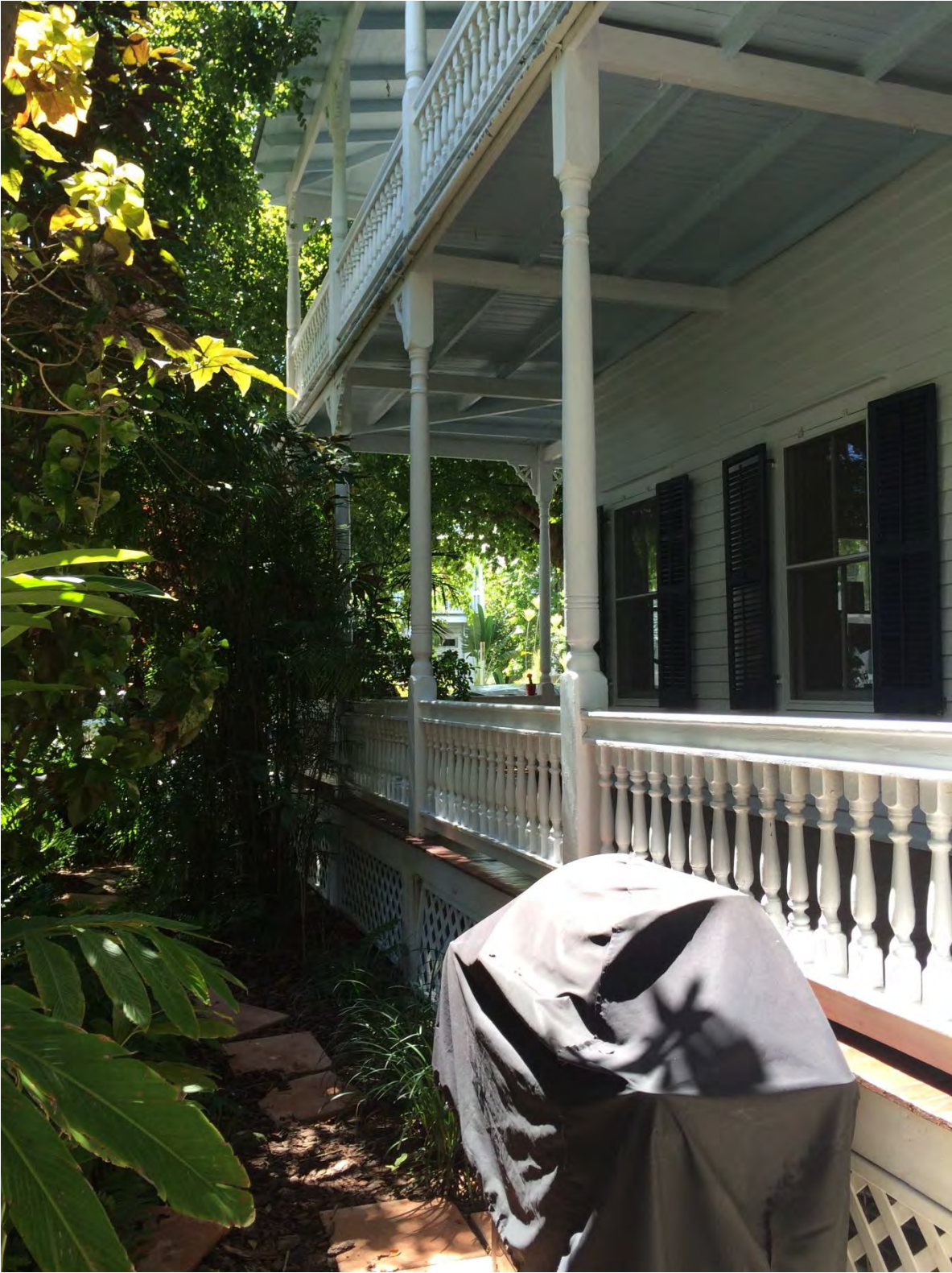
925 FLEMING STREET: SIDE OF HOUSE
