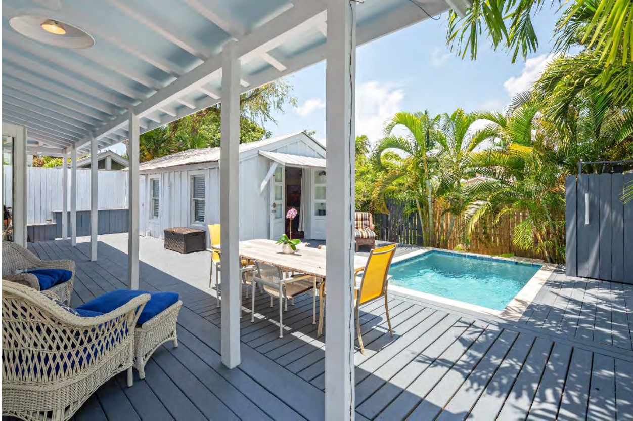
View of accessory structure.
