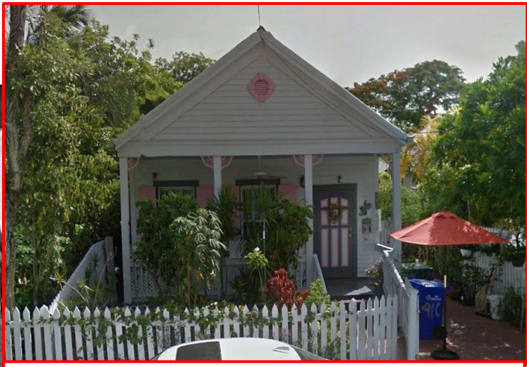
910 Thomas Street. "Exhibit 2" labels it as 1.5-stories, though it appears to be 1-story.
