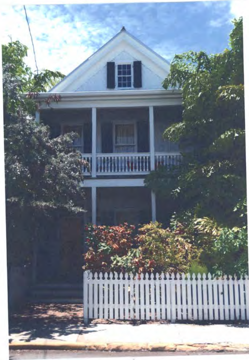
FRONT OF MAH HOUSE (OLYIA ST.)
