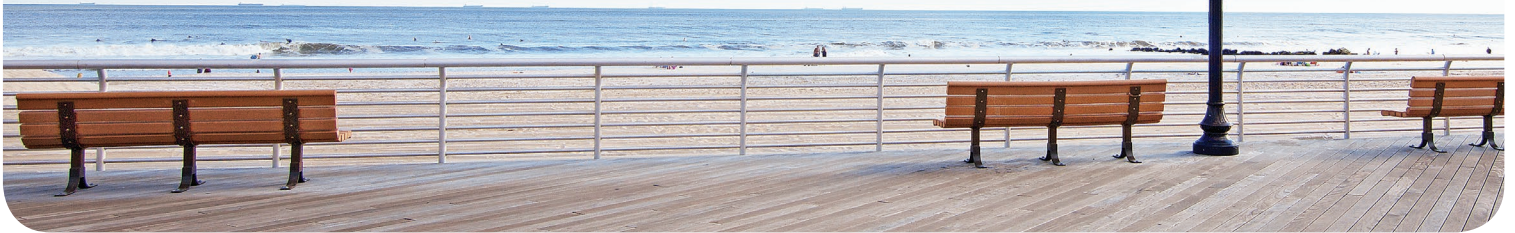
Long Beach Boardwalk – Long Island, NY Reconstruction after Hurricane Sandy
