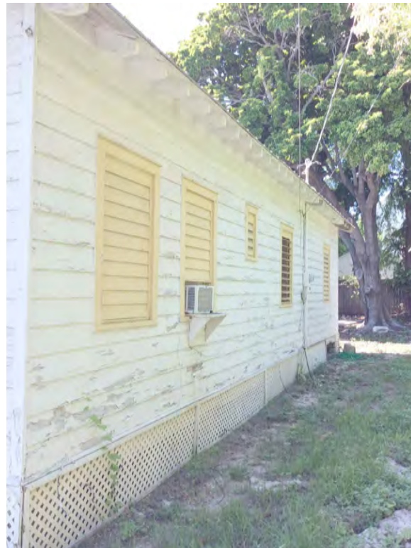
FIGURE 4 RIGHT SIDE VIEW OF HOUSE
