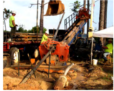
Horizontal Oxygen Infusion Well
