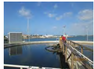
Through the execution of the current General engineering Services Contract with the City of Key West, the Black & Veatch key team members have already become familiar with the current operations and needs at the Wastewater Treatment Plant.
