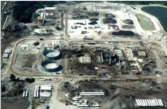
Civil/Site development for a Tampa Bay Water facility.
