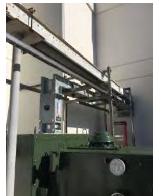
BCWWS Electrical Load Center no. 1 – Transformer replacement Construction Project
