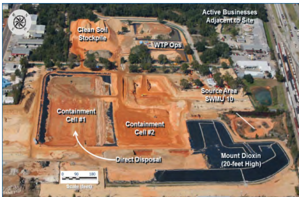
Escambia OU1 Soil Stabilization/Containment
