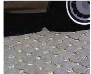
Green solutions, such as the porous pavement pictured above, can provide benefits to multiple stakeholder groups.
