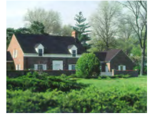
Pump station designed by Black & Veatch to resemble a private residence.
