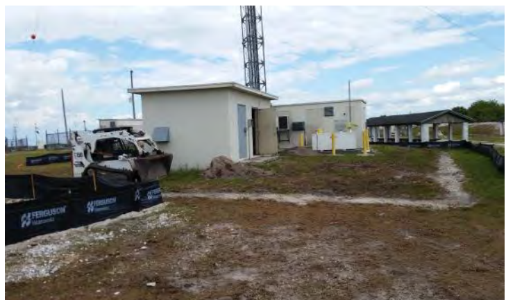
IT Shelter Replacement Construction – New SCADA Building
