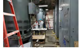
BCWWS Outfall Pump Station – Shorting Contactor Replacement Construction Project
