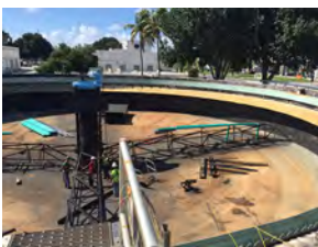
BCWWS Clarifier – Clarifier A3 Rehabilitation Construction Project
