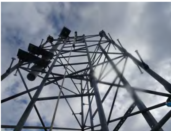
S-127 Command and Control Center North Shore Path Automation Construction Project – Microwave Tower
