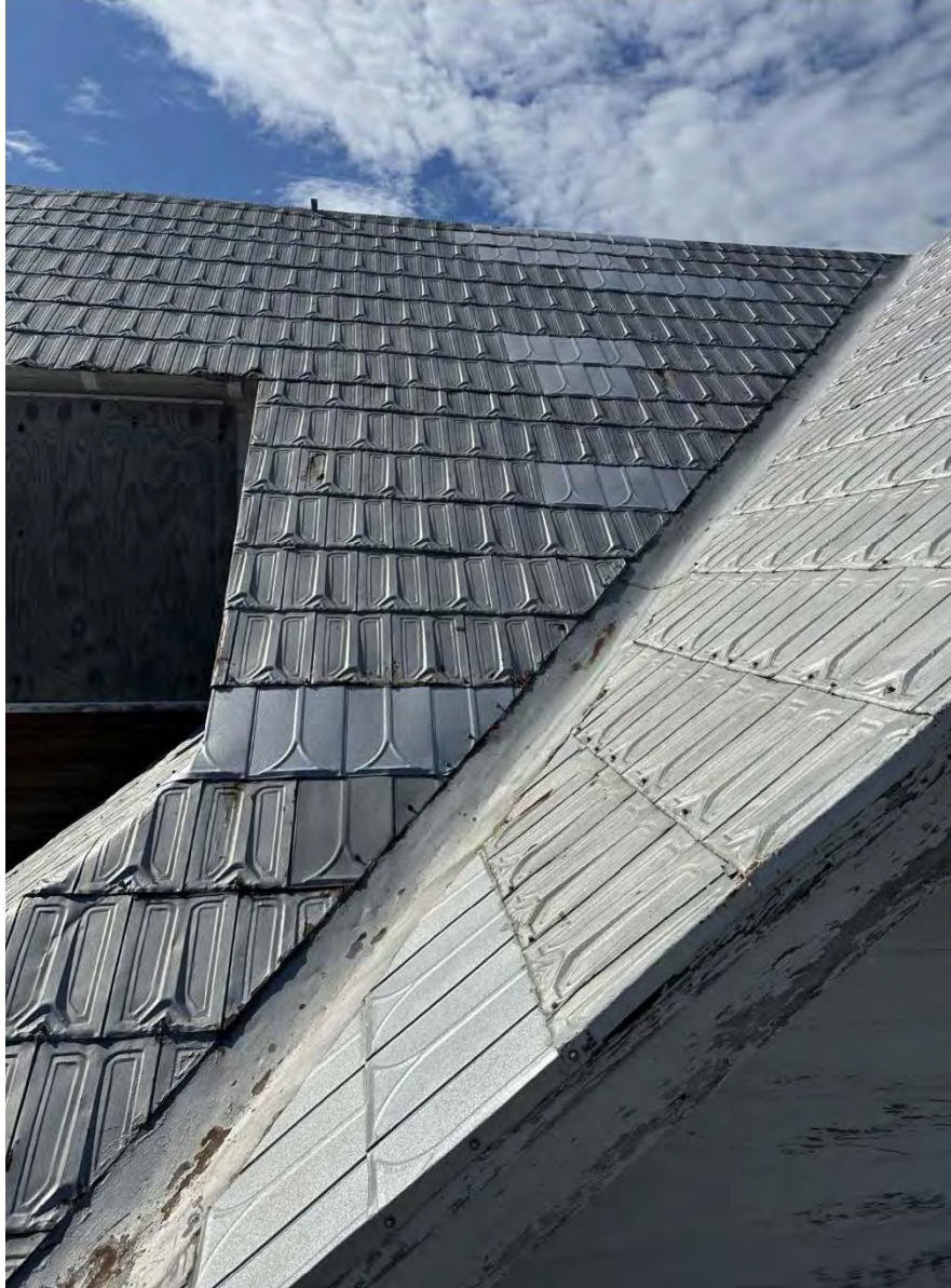
Detail of existing roofing. Photograph provided by applicant.
