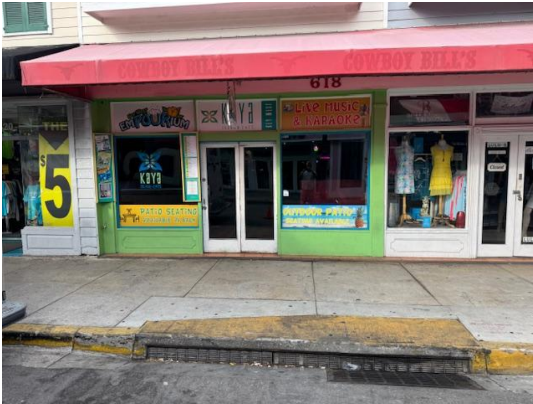
Photograph of existing storefront system.
