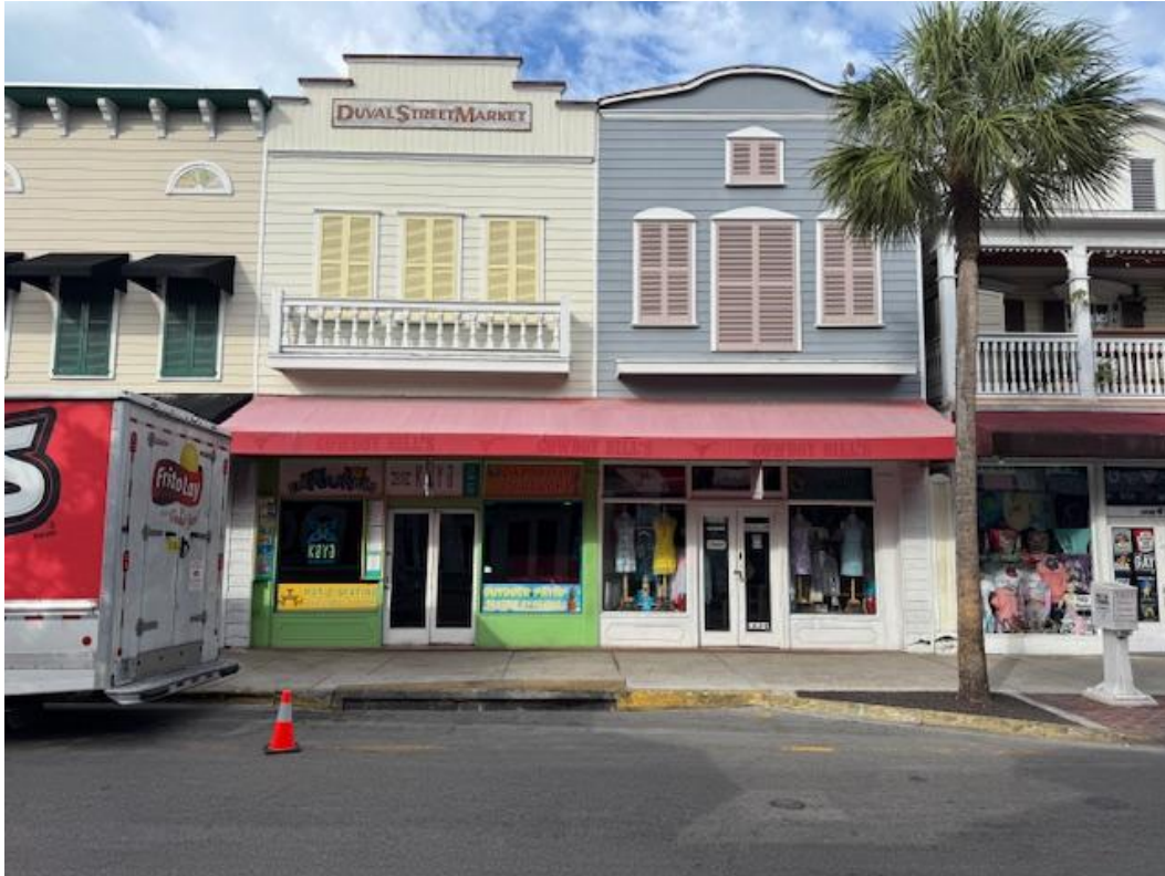
Photograph of 618 Duval and adjacent structure.
