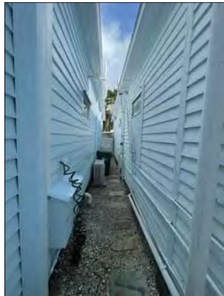
8 LOOKING SOUTH FROM WEST SIDE YARD
