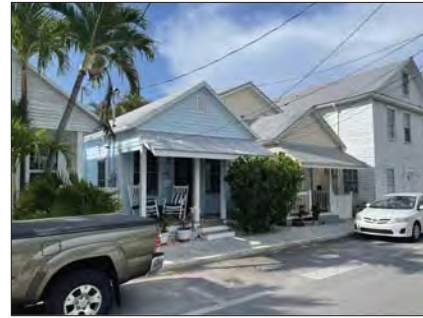
3 LOOKING SOUTHWEST ON OLIVIA STREET
