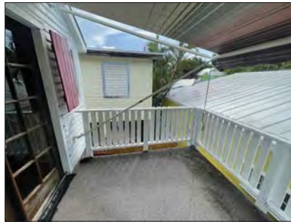
9 LOOKING EAST AND SOUTH FROM REAR BALCONY
