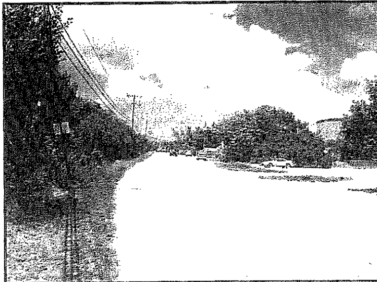
Street Scene Looking Northeasterly Along College Road
