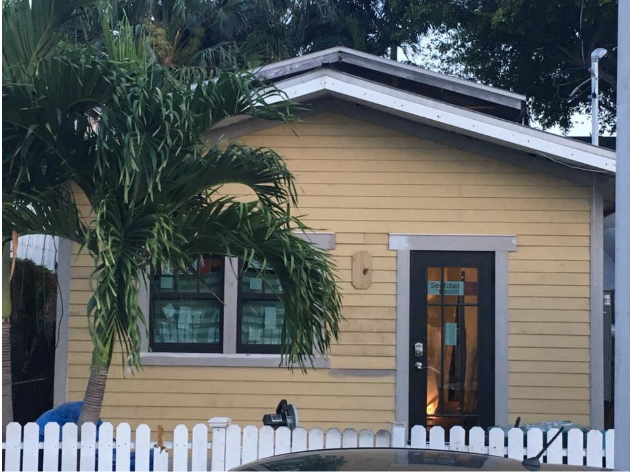
904 Olivia front elevation (in progress renovation)
