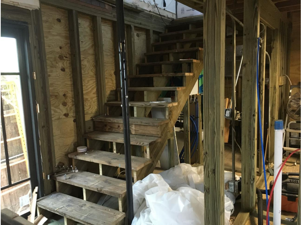
904 Olivia interior stairs (in progress renovation)
