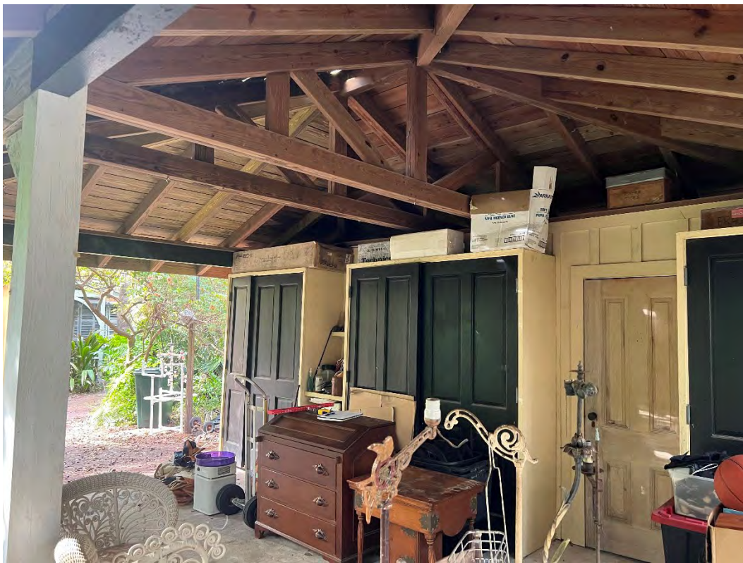
Existing Carport – Enclosed Storage and Laundry on West Side
