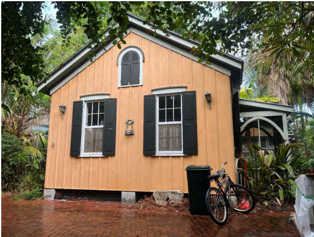
Main House - North
