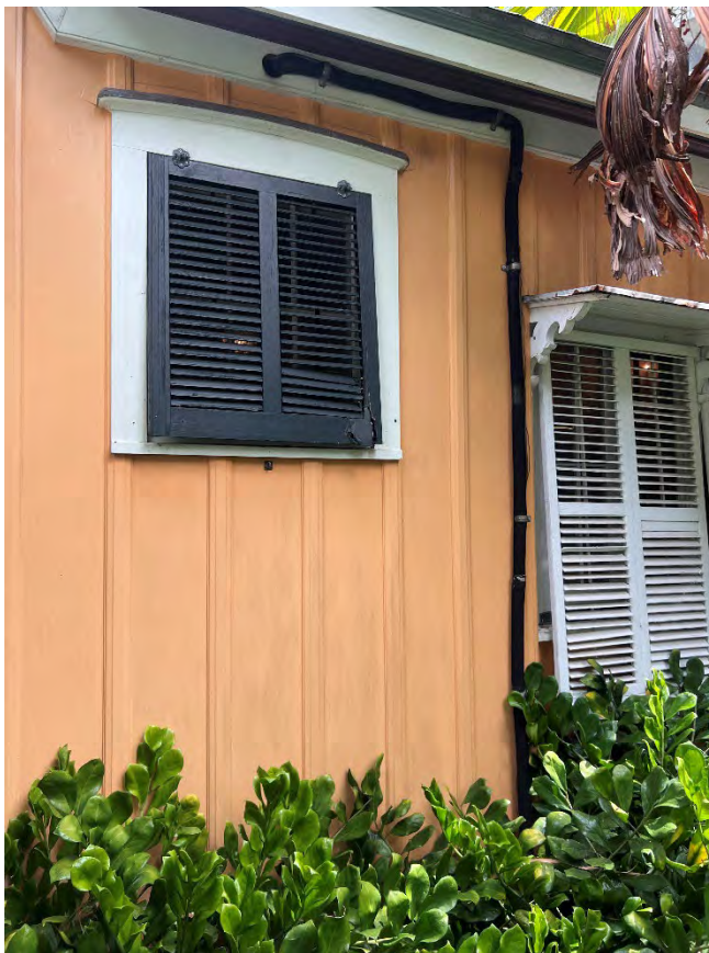
Existing 6-Lite High Window at Main House with Shutter
