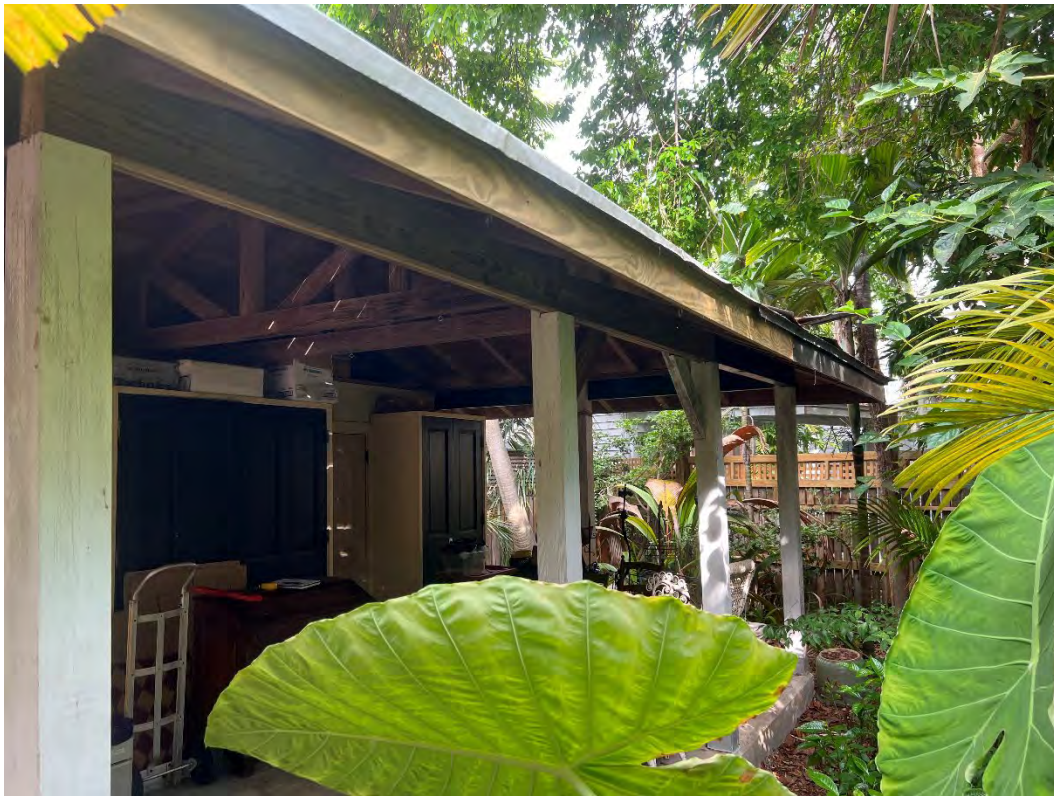
Existing Carport - East
