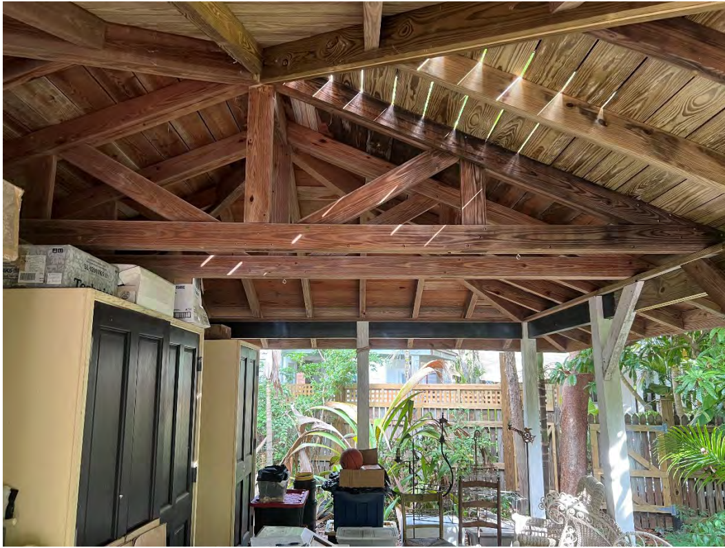
Existing Carport Roof Structure
