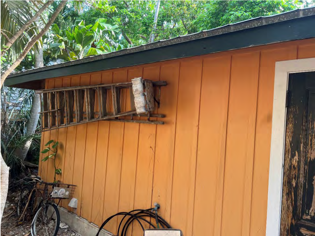
Existing Carport – Enclosed West Side
