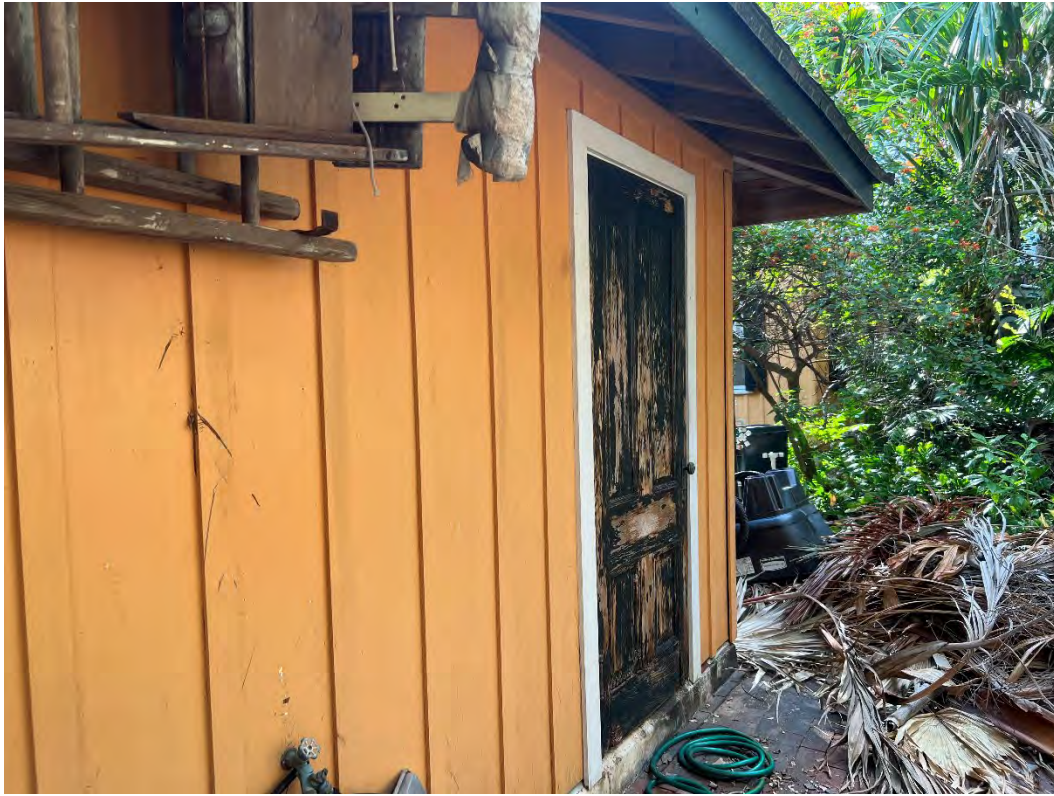
Existing Carport - West
