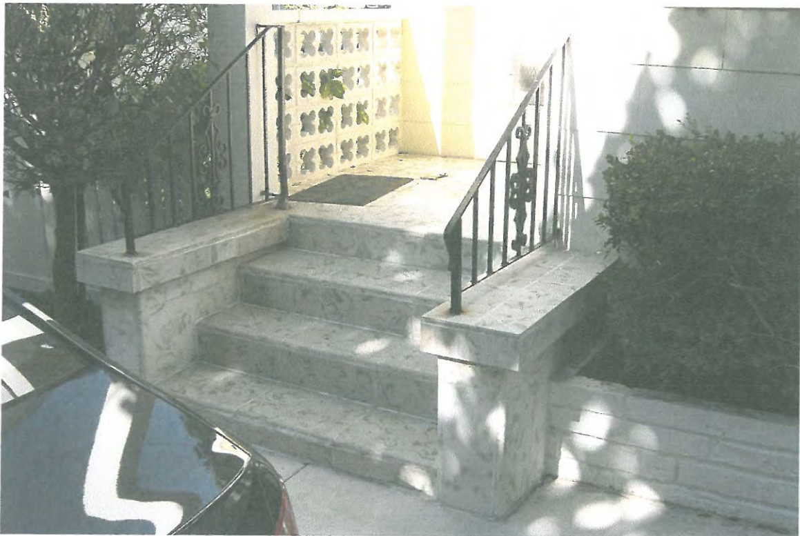
FRONT PORCH STEPS 1117 STUMP LN.
