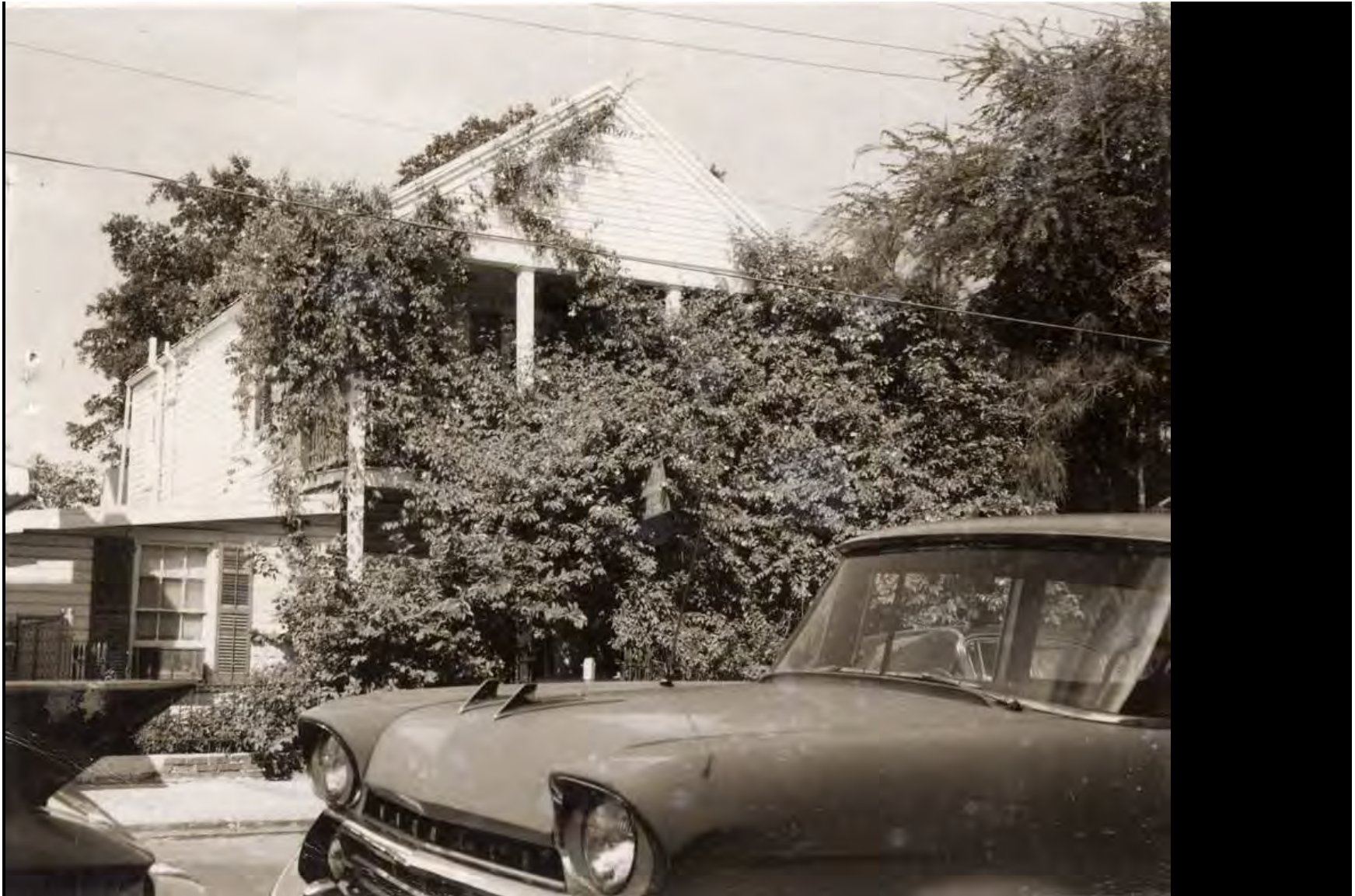
Photo taken by Property Appraiser's office ca.1965; 217 Duval St.; built 1889. Monroe County Library
