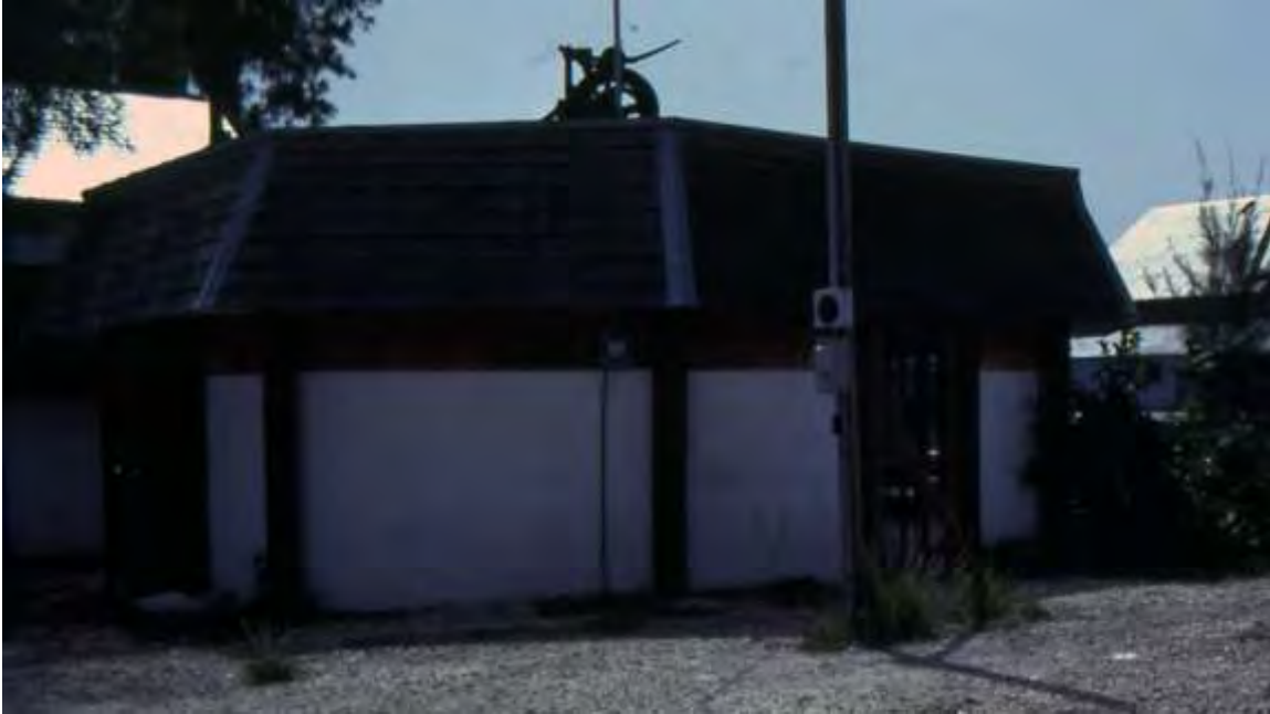
West cable hut circa 1984 looking southeast. East cable hut and Hospitality house towards the left side of the photograph. Monroe County Library
