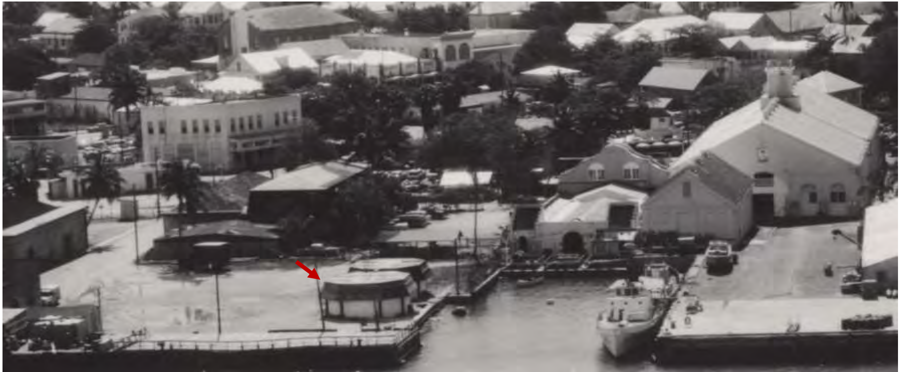
Aerial photograph circa 1958. Both Cable huts still as utilitarian tanks at the Mallory Dock.
