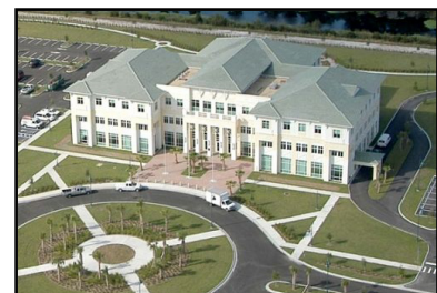
North Port City Hall
