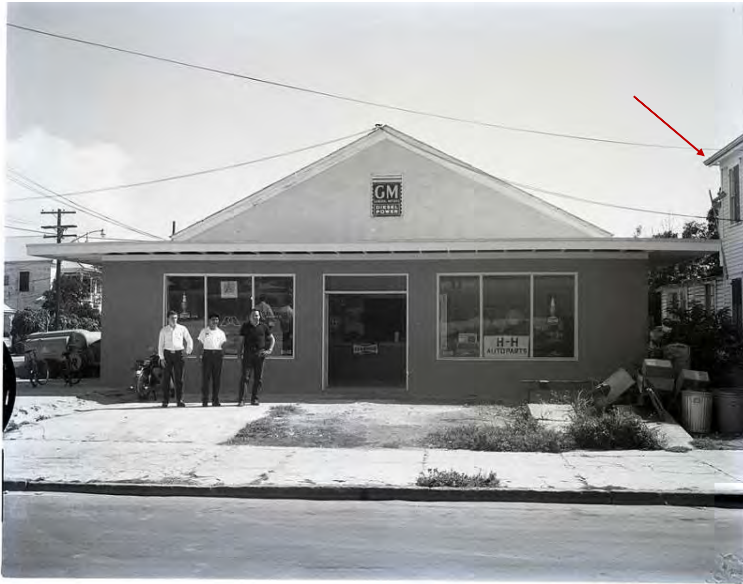
726 Caroline Street in 1966. House under review towards the right side. Monroe County Library.
