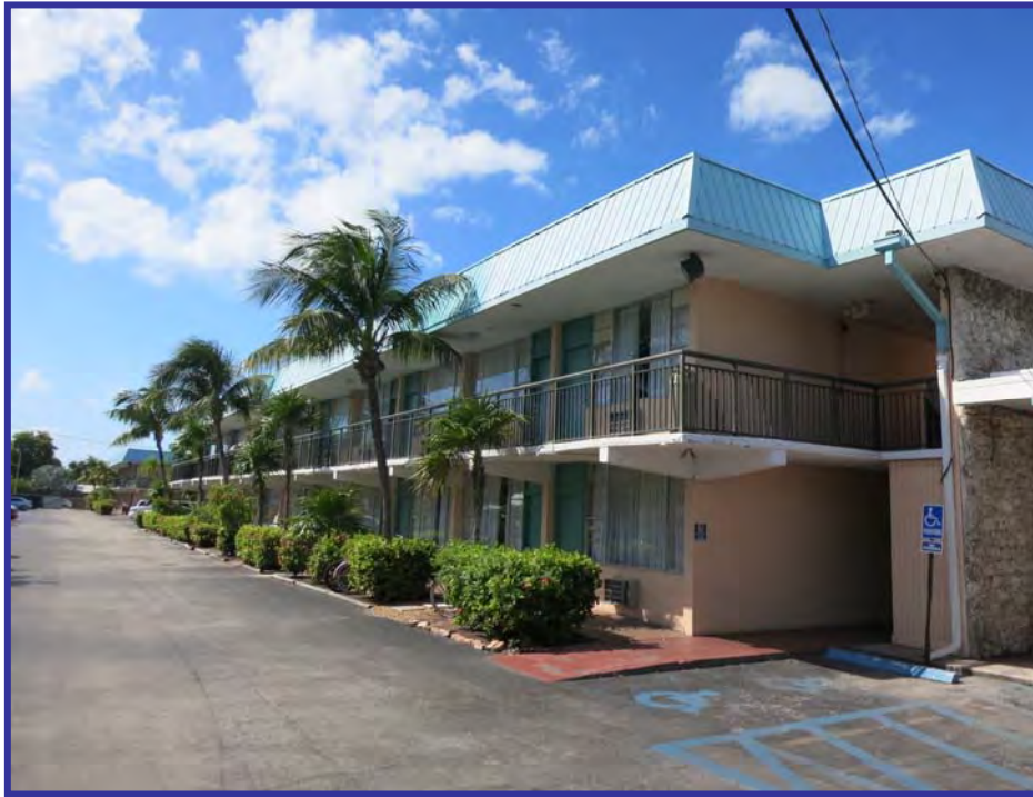
View looking southwest
