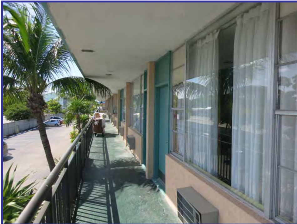
View of the 2nd floor covered walkway
