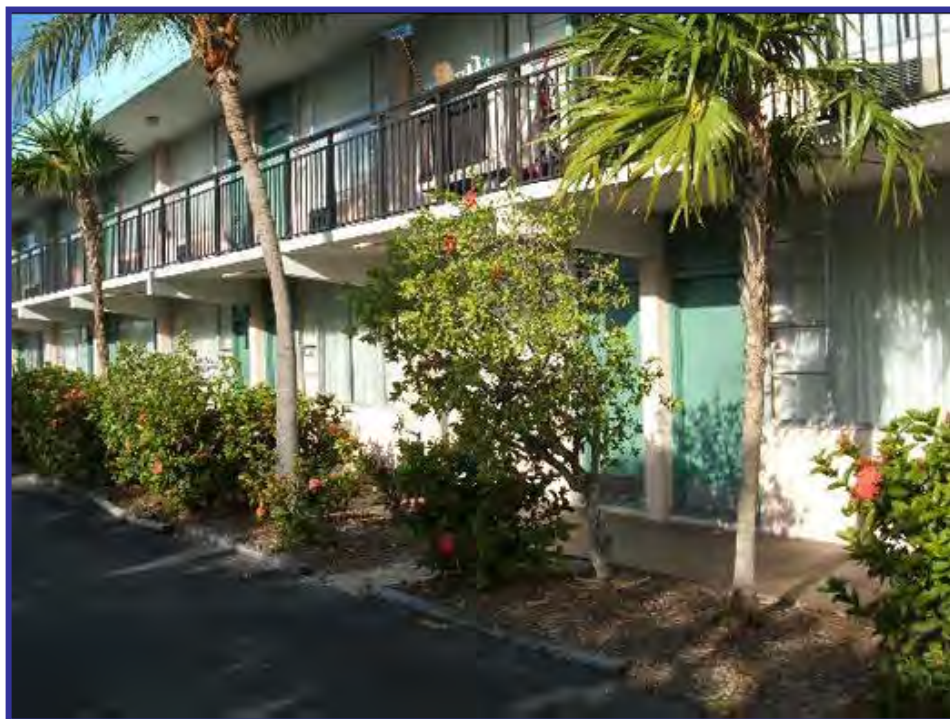
Close-up view of southeast side of the building
