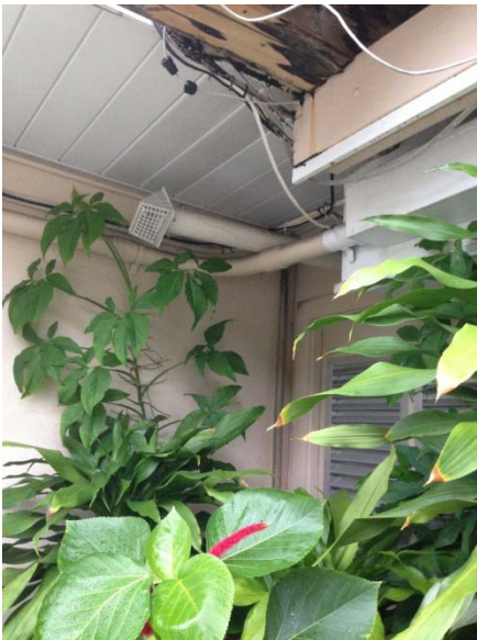
Photograph 9 of what appears to be an end of the line cleanout for the L shaped structure. The pipe appears to be made of cast iron and does not have a clean out box around it.
