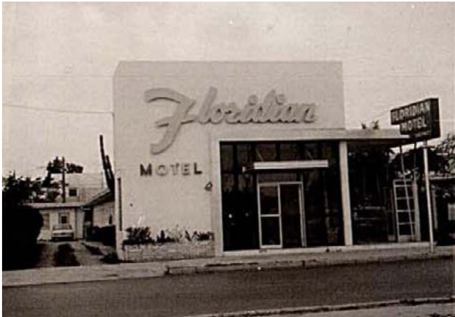
Exhibit A – Original front façade on Simonton Street
