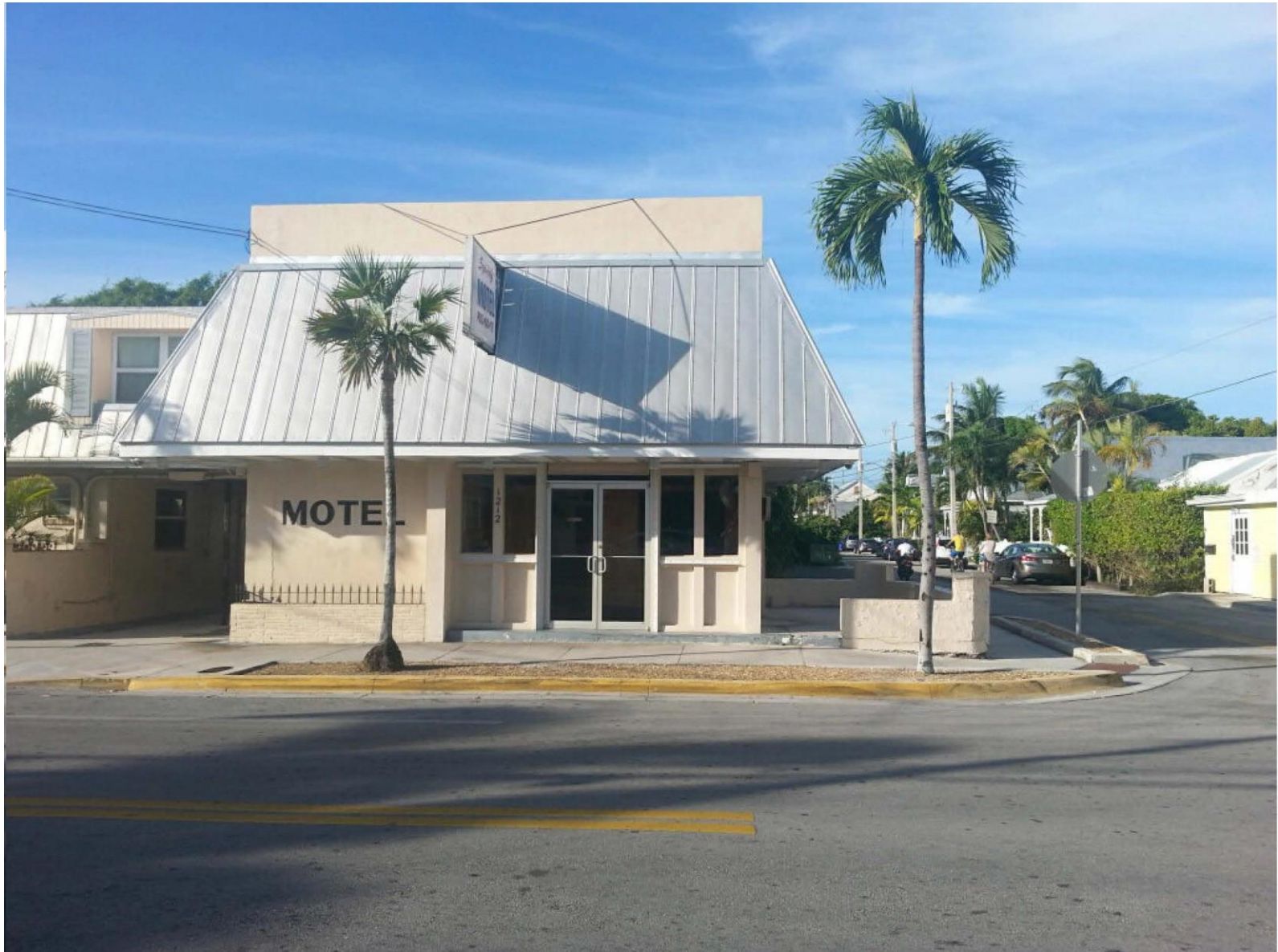
The Florida Motel today. Other than the parapet wall, all other character defining features are gone.
