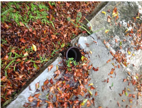
Photograph 8 of the exterior of the L shaped building on Louisa Street. Note the egress window blocked by the air conditioning unit. It appears that the units had an egress door to Louisa Street that was in-filled at some point.
