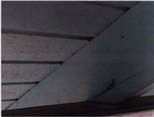
(Pic.12) Upstairs bar roof rafters (No visible roof uplift connections)
