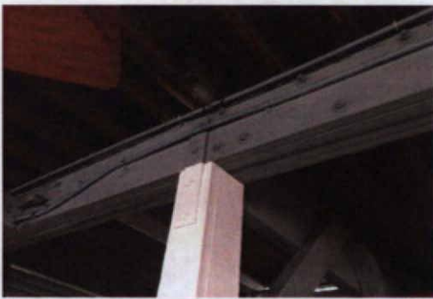
(Pic.2) Typical Interior Roof Framing and Support
