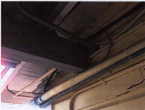
(Pic.8) Inadequate beam support at walkway canopy structure
