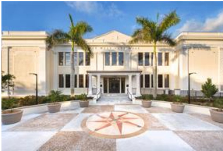
Figure 1 # 1. Front Entrance - retaining wall
