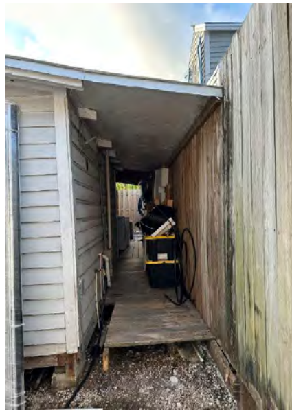
Existing rear elevation of side covered porch under review.
