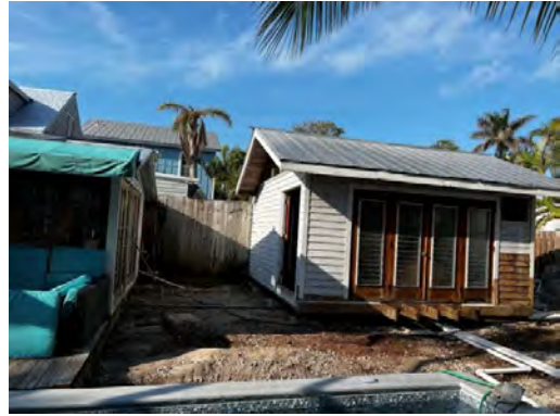
Side of structure under review, existing.
