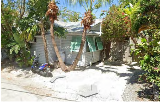
Front of structure under review, existing.
