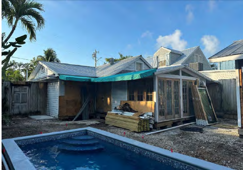
Rear elevation of primary structure under review and pool.
